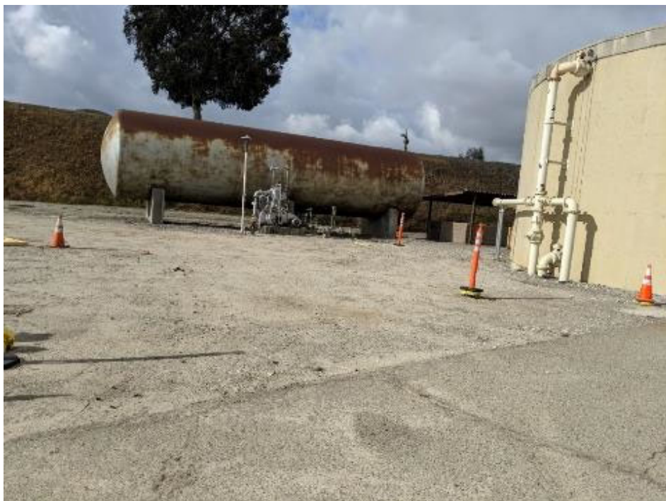
Photo 2. Planned location for Pump Station and Centrate Equalization Tank, looking south. Note area is developed and devoid of vegetation.
