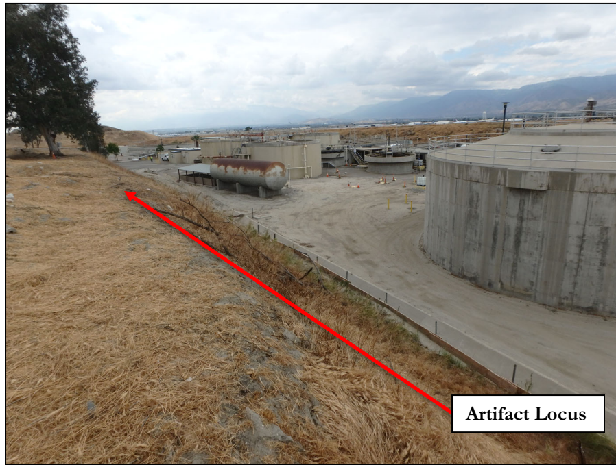
Figure 6. Overview of WWTP, Digester Tank 2 and Reserve Digester and Methane Gas Storage Tank (1972), looking northeast. Note artifact locus on terrace edge above WWTP, on left side of image.
