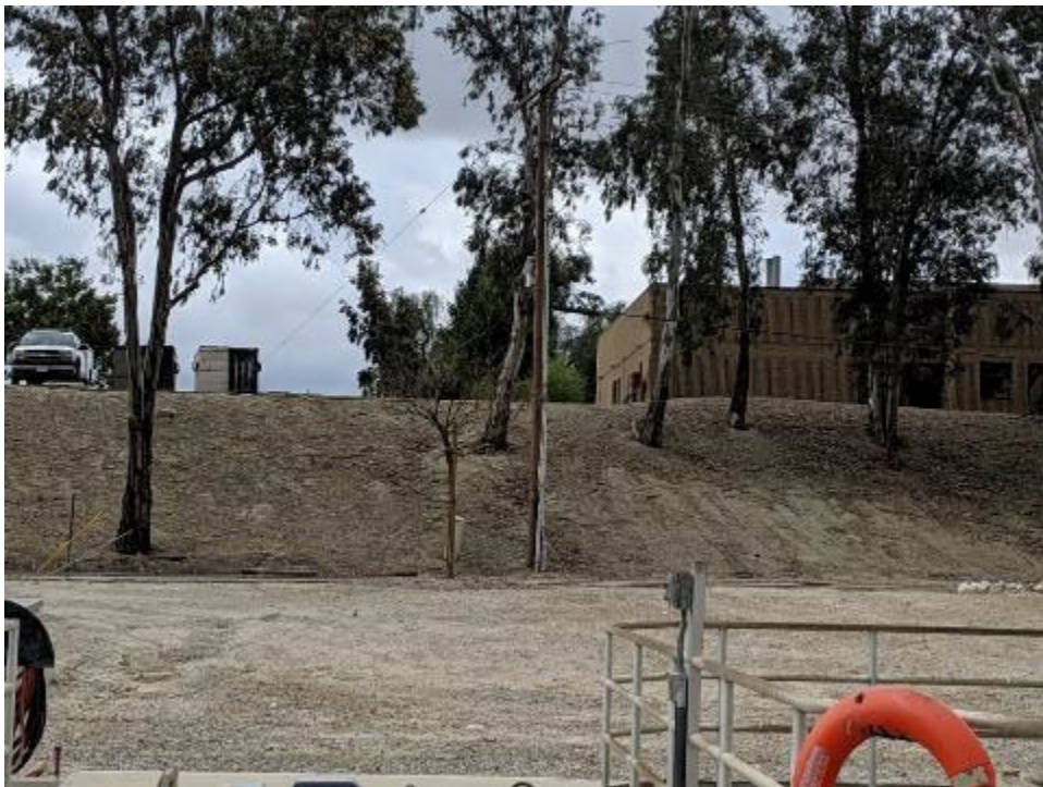
Photo 22. Looking north toward main office building. Areas around building are planned for landscaping improvements. A patio and walkway to the plant operations area are planned on the north side of the building.
