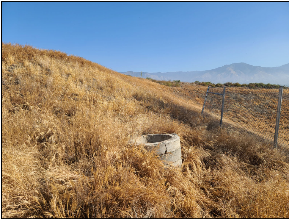
Figure 14. Overview of Feature 39, Water Fitting Access Structure, looking north.
