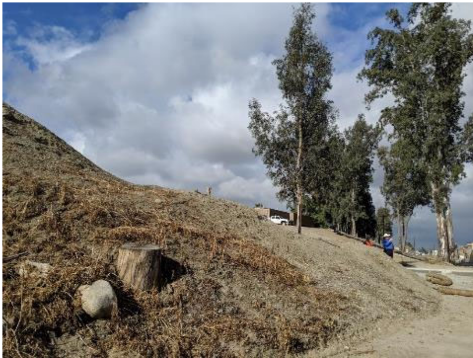
Photo 4. Planned location for SWBD-M Electrical Building, looking southeast. This site is dominated with ruderal vegetation and planted eucalyptus and pine trees.
