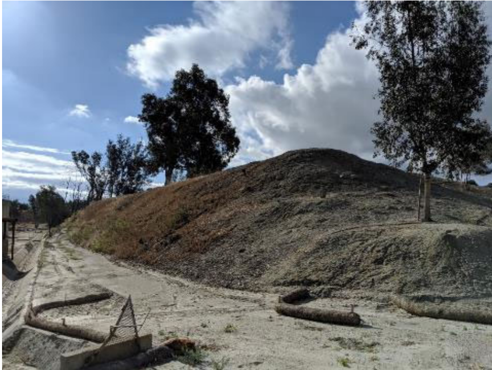
Photo 17. Looking southeast toward hillside planned for slope protection landscaping improvements.
