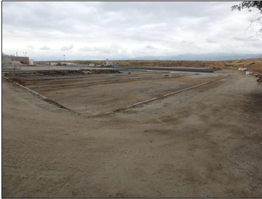
Figure 10. Overview of Drying Beds (1972), looking northwest.
