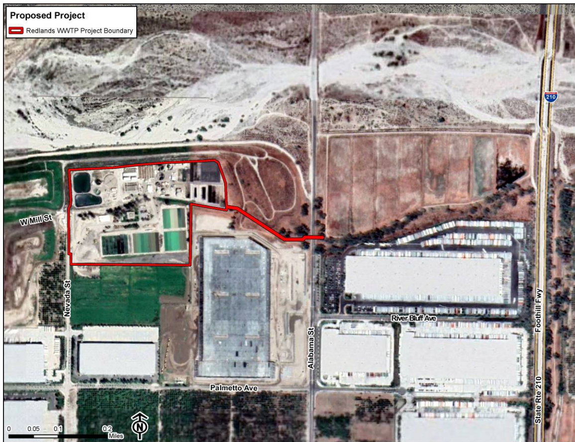
Figure 2. Aerial Photograph of Existing WWTP
