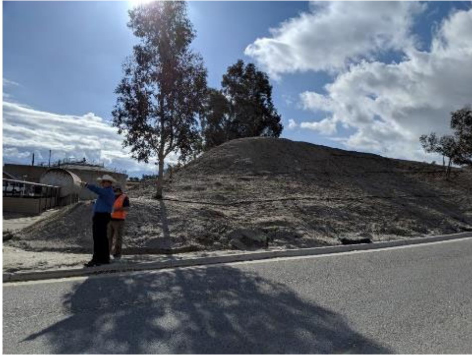
Photo 3. Planned location for SWBD-M Electrical Building, looking southwest. This site was formerly a farmer dump site, and old cans and materials may be buried underneath. Vegetation at this location is mainly ruderal with planted eucalyptus and pine.
