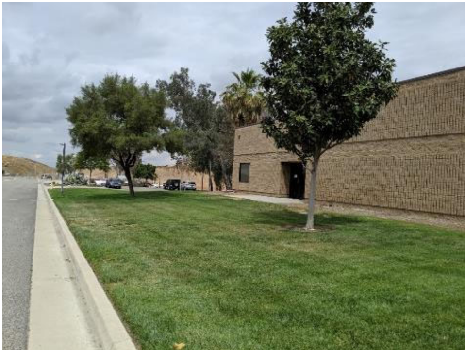
Photo 24. Looking at south side of building where walkway and patio improvements are planned.
