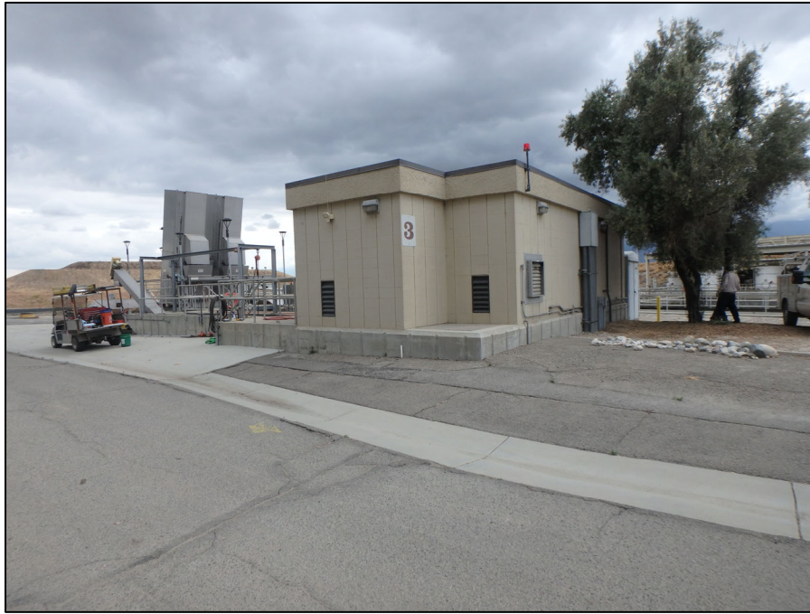
Figure 12. Overview of Building 3 (Headworks Building) and Headworks (1972), looking northwest.
