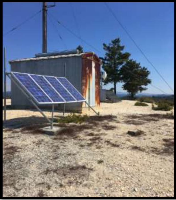
Photo 5: Existing facilities at Chalk Mountain.
