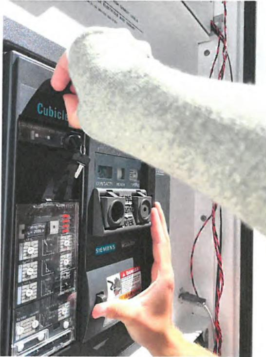
3. Insert the lock, lock it, and secure the AC circuit breaker:
