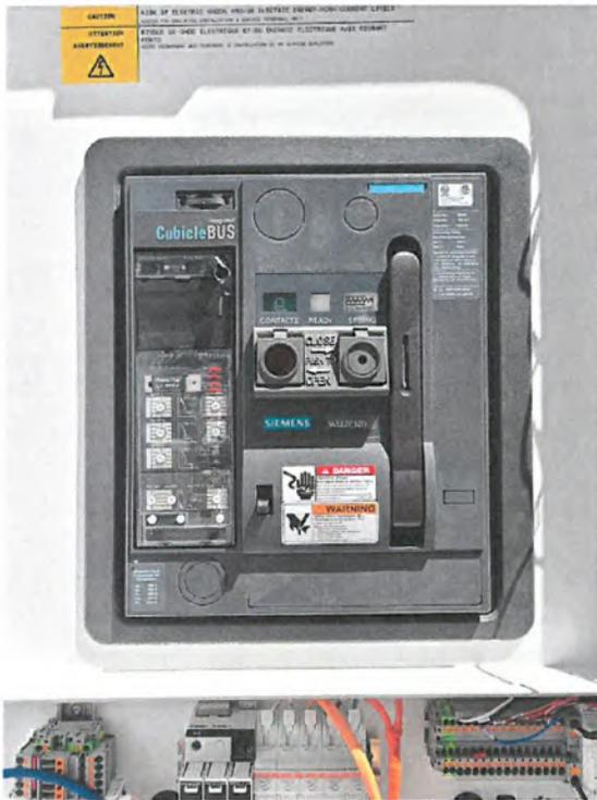
The circuit breaker is shipped with pre-configured general trip settings that must be changed upon arrival through the Electronic Trip Unit (ETU). The ETU has configurable settings for Long-time overcurrent protection (L), Short-time delayed overcurrent protection (S), Instantaneous Overcurrent Protection (I), Ground Fault Protection (G), and other features provided below. The Engineer of Record is responsible for the configuration of the ETU settings for system protection and proper operation.
