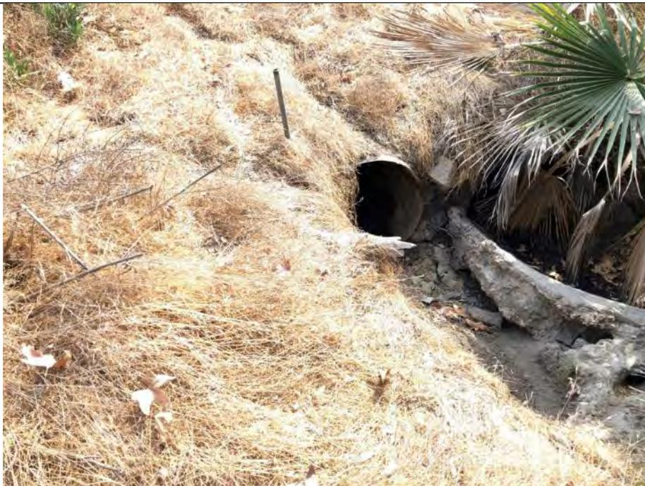
**Photo 4:** View of pipe culvert beneath on-site dirt road.
