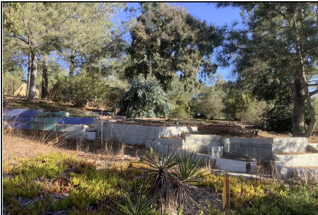
PHOTOGRAPH 2 Overview of Foundations, Looking Northeast
