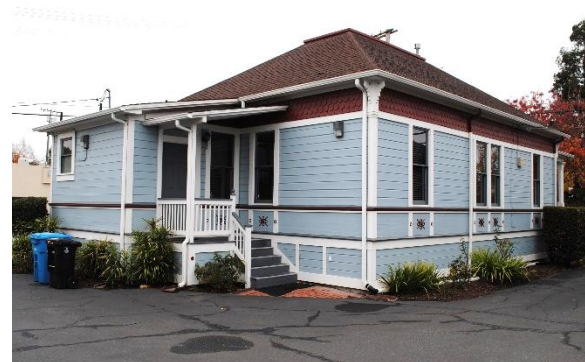
Figure 7. Oblique view of rear (west) and south façades, looking northeast.
