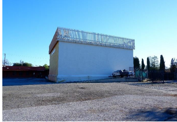
Figure 40. North and west facades, looking southeast.
