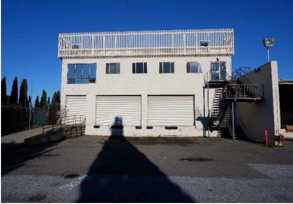
Figure 39. South façade of the 1980 warehouse-office building, looking north.
