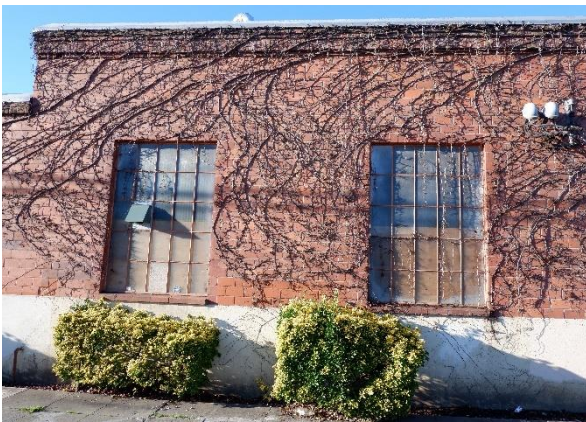
Figure 21. Typical windows at the 1931 garage, looking west.
