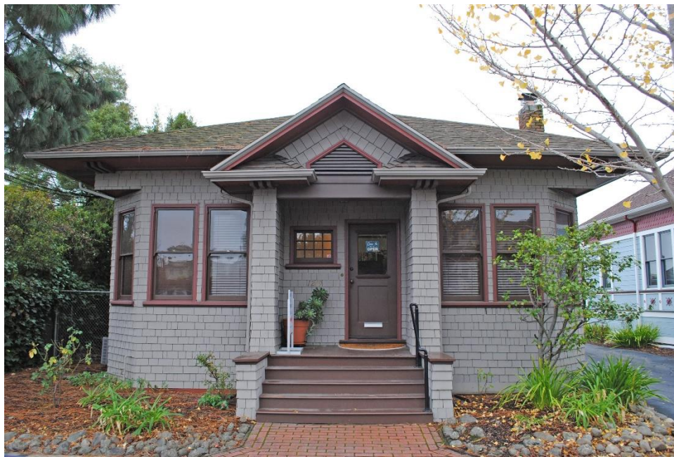
Figure 8. Primary (east) façade of 1219 Arguello Street.
