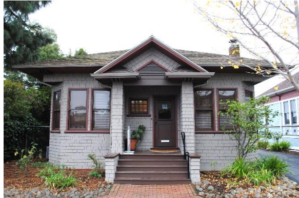
Figure 4. Primary (east) façade of 1219 Arguello Street.
