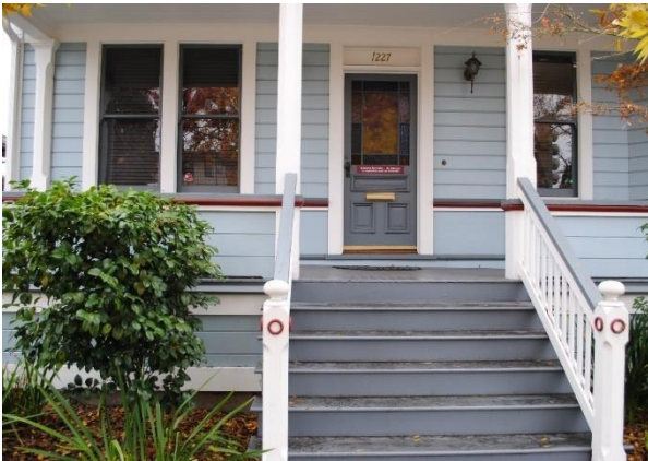
Figure 4. Steps to front entry porch.
