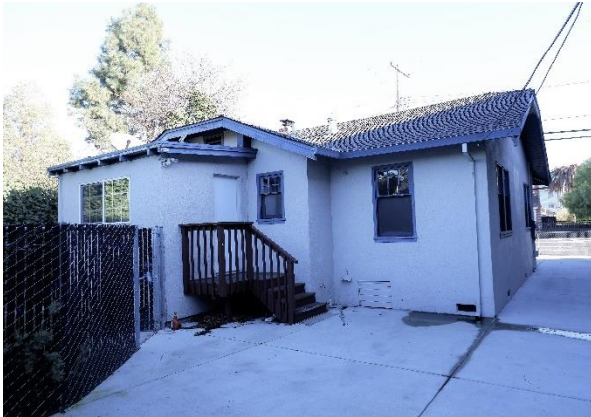
Figure 15. Rear (west) and south facades, looking northeast.
