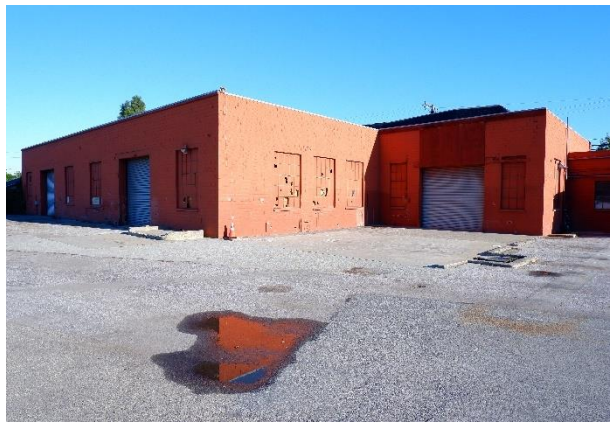
Figure 22. Rear (west) and south facades of the 1931 garage, looking northeast.
