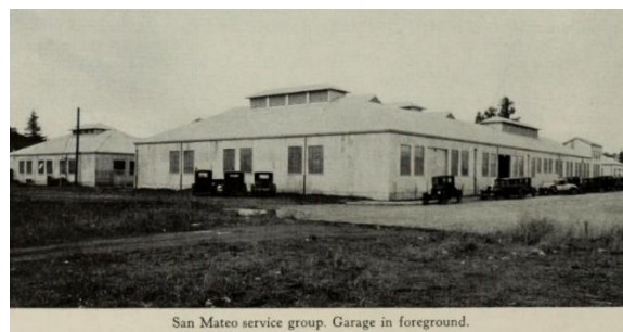
Figure 44. PG&E's San Mateo Service Group, with more industrial corrugated metal exterior, ca. 1933. Source: Pacific Service Magazine (1933).
