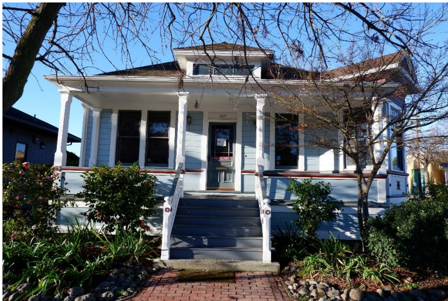
Figure 3. Primary (east) façade of 1227 Arguello Street.
