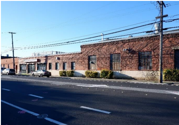
Figure 18. 1125 Arguello Street, looking southwest.
