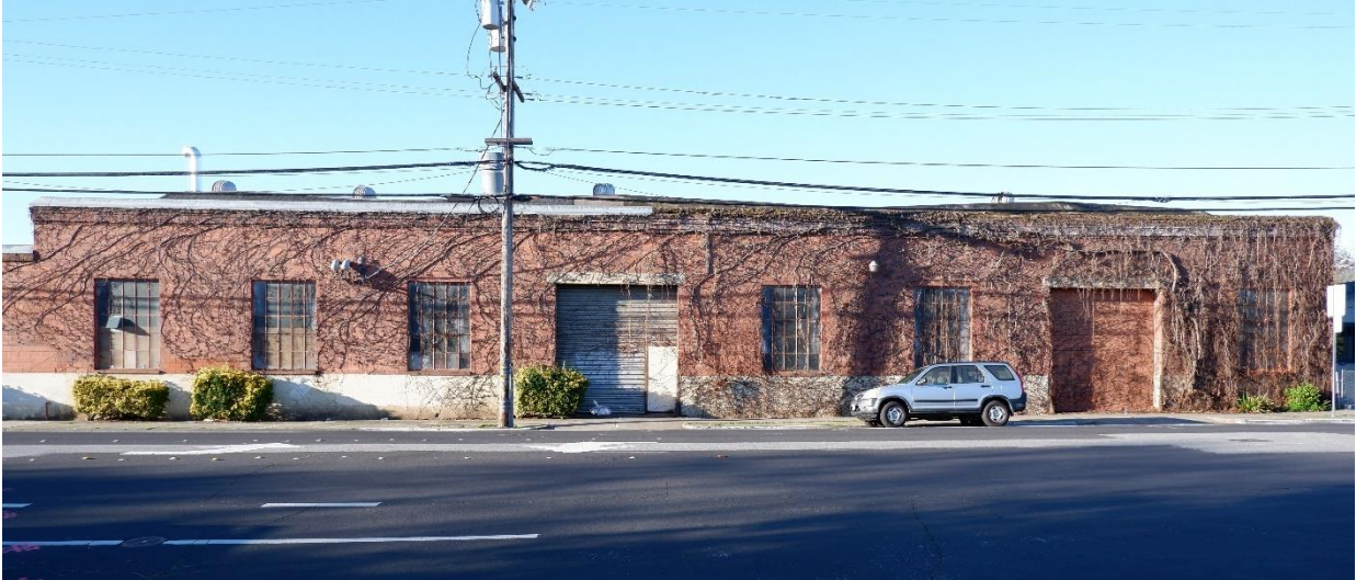
Figure 20. Primary (east) façade of the 1931 garage, looking west.
