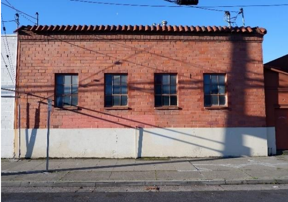
Figure 31. East façade of the 1931 warehouse at 1111 Arguello Street, looking west.
