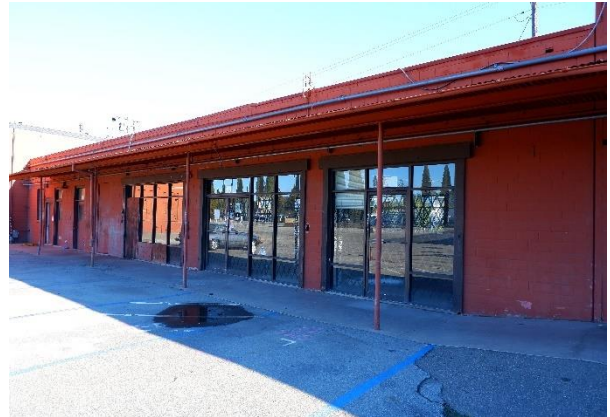
Figure 27. Rear façade of the 1931 office building, looking northeast.
