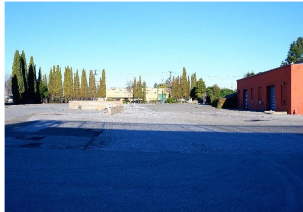
Figure 19. Rear service yar, looking north toward Whipple Avenue.
