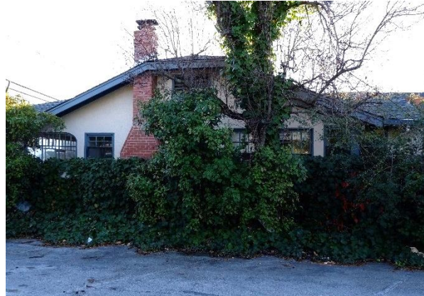
Figure 16. North façade, looking south.
