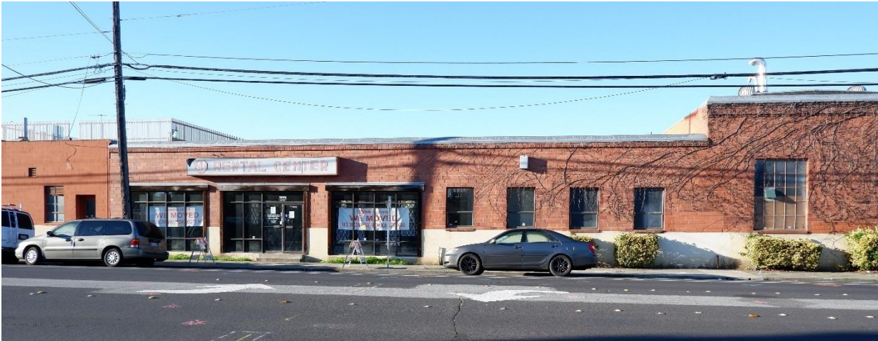
Figure 23. Primary (east) façade of the 1931 office building, looking west.
