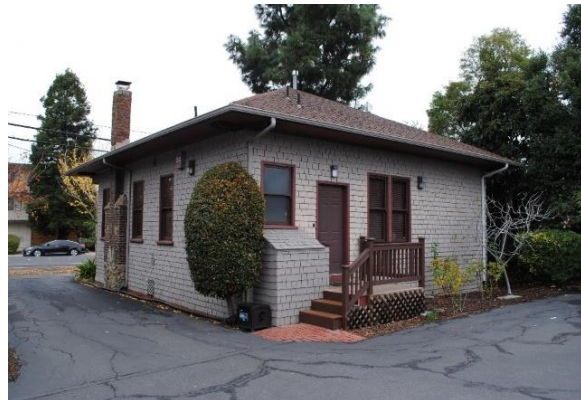
Figure 10. Oblique view of north and rear (west) façades, looking southeast.
