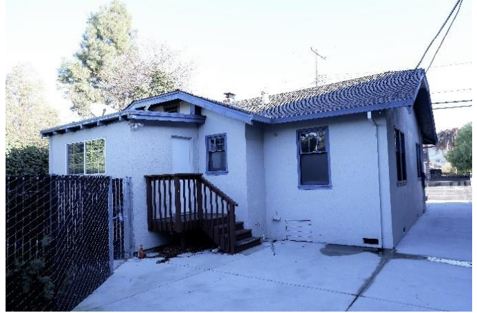
Figure 2. Rear (west) and south facades, looking northeast.
