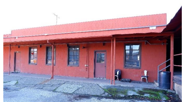
Figure 29. Rear (west) façade of the 1959 office building addition, looking northeast.
