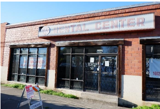
Figure 24. Doorway in the central storefront at 1931 office building, looking southwest.
