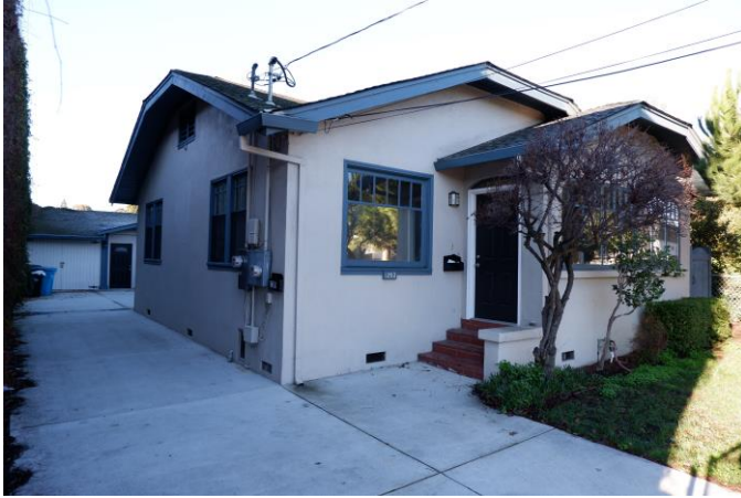
Figure 1. Primary (east) and south facades, looking northwest.
