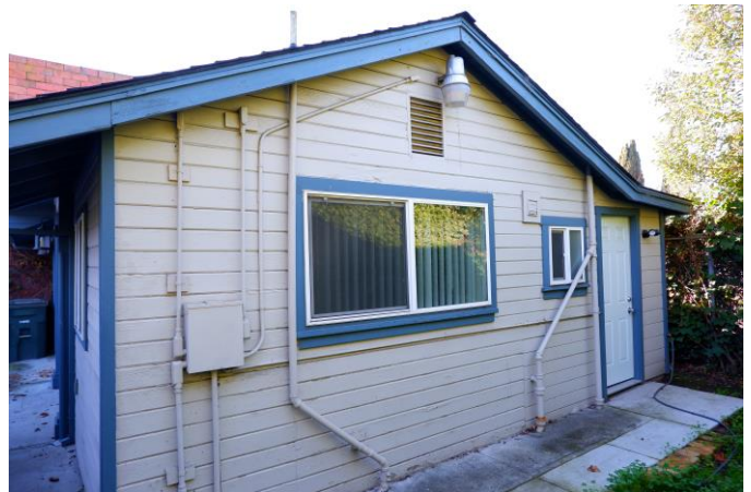
Figure 4. North façade of the detached rear garage and ADU, looking southwest.
