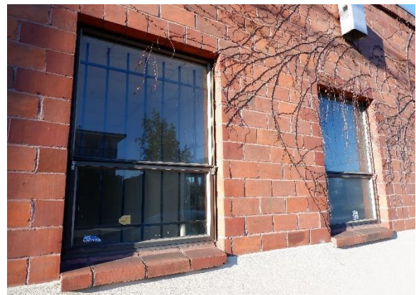
Figure 25. Replacement aluminum sash windows in original openings, looking northwest.
