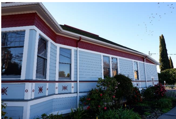
Figure 6. View of north façade.
