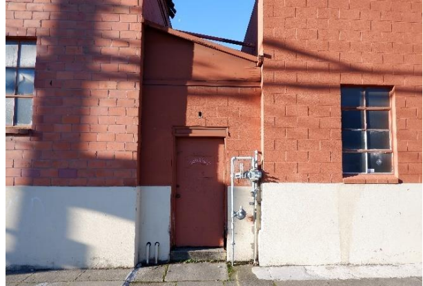
Figure 32. East wall partially enclosing the loading dock (center) on the north side of the 1931 warehouse (left).
