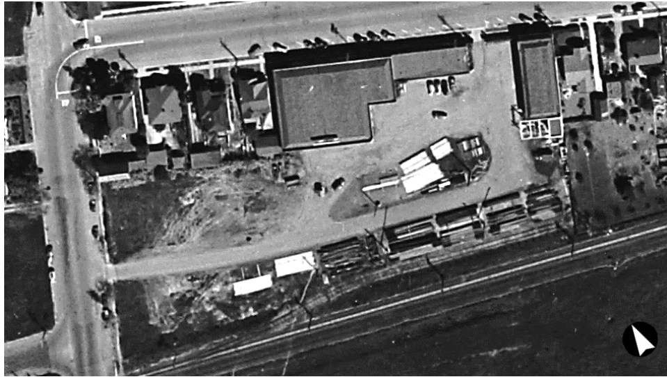
Figure 53. From left to right, 1229, 1219, 1209, and 1203 Arguello Street and the PG&E Redwood City Service Group at 1111-1125 Arguello Street, 1941. Source: Flight C-6660, Frame 311, Fairchild Aerial Surveys, UC Santa Barbara FrameFinder.
