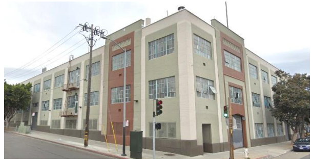
Figure 46. PG&E San Francisco (Mission) Service Group facility at 3235 18 th Street. Source: Google Street View, April 2019.
