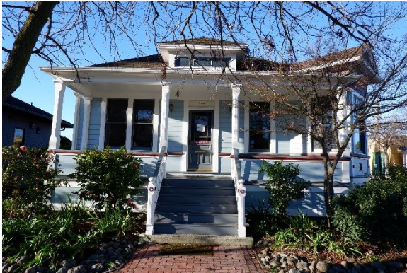
Figure 3. Primary (east) façade of 1227 Arguello Street.
