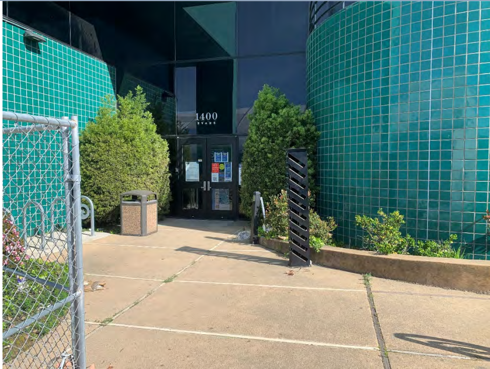
Entrance to main building at Target Site
