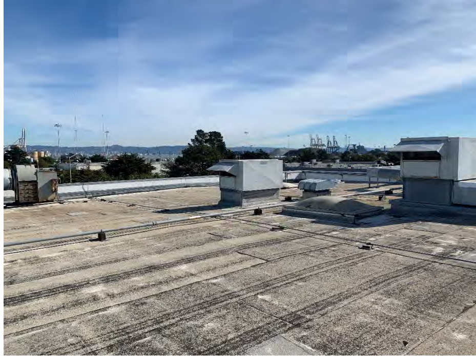
Roof of building on Target Property looking east.
