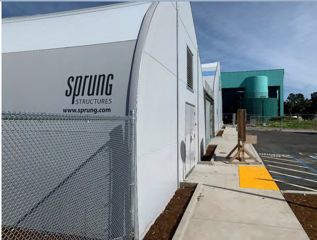
Temporary structures in southern portion of Target Site and entrance to main building.
