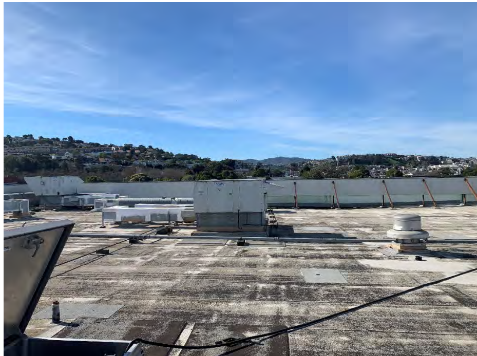
Roof of building on Target Property looking south
