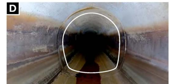
Tunneled, Cast-in-Place Pipe (Hoseshoe Shaped)
