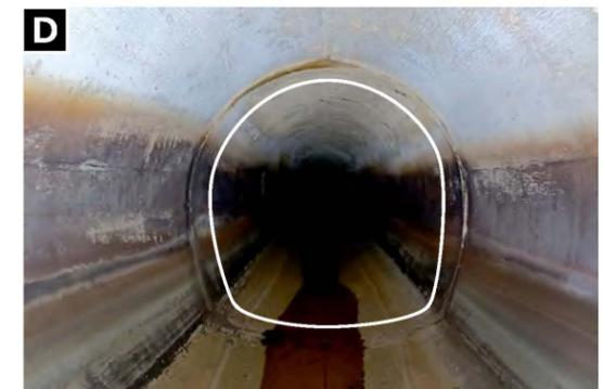
**Tunneled, Cast-in-Place Pipe (Hoseshoe Shaped) 20-ft Sections; Cross-Sectional Area = 29.9 SF**
