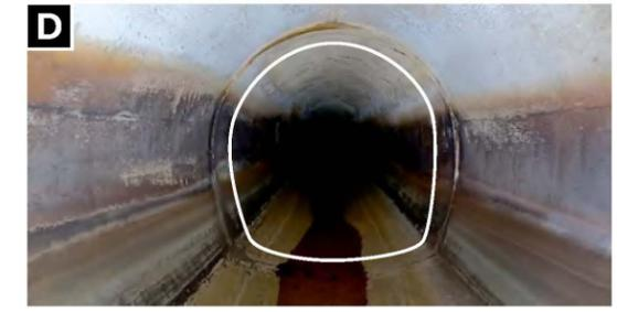
**Tunnelled, Cast-in-Place Pipe (Horseshoe Shaped)**
