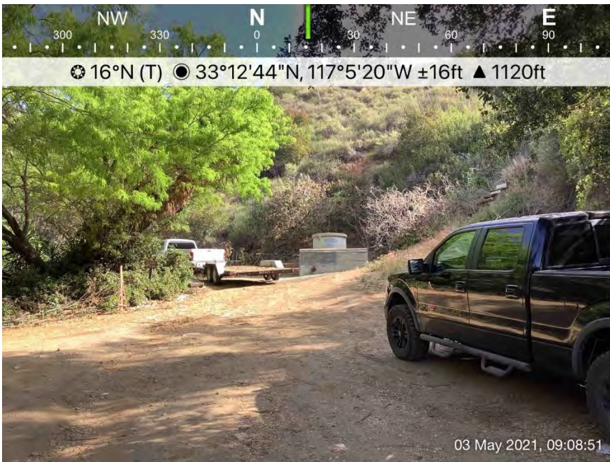
Photo 20: The potential work area within Study Area 7 is centered around the downstream Oat Hills Tunnel bifurcation structure. The structure is surrounded by non-native woodland, urban/developed land, disturbed habitat and coastal sage scrub.
