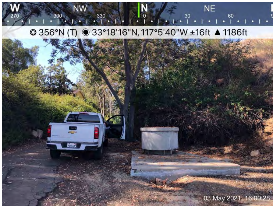
Photo 2: The southern potential work area within Study Area 1 is centered around the downstream Lilac Tunnel bifurcation structure. The structure and potential work area is surrounded by non-native woodland, non-native grassland, disturbed habitat and orchards.
