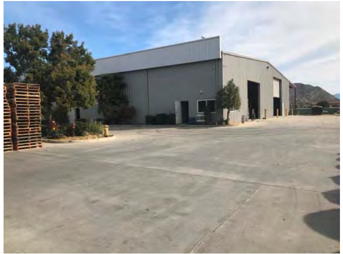
4. View northeast of the Site production warehouse.
