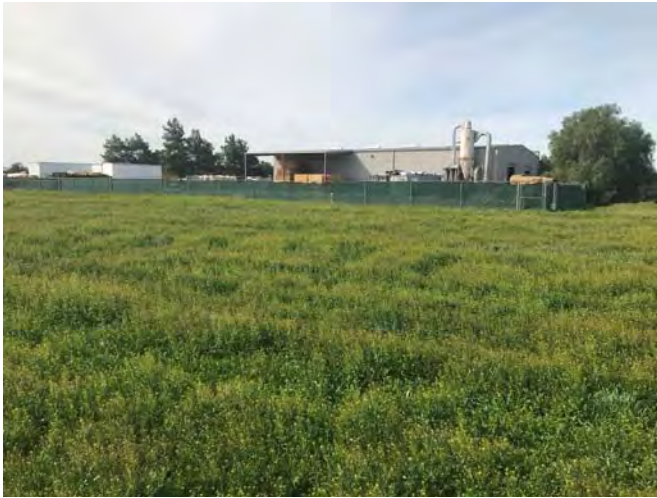
13. View west of the Site facility.
