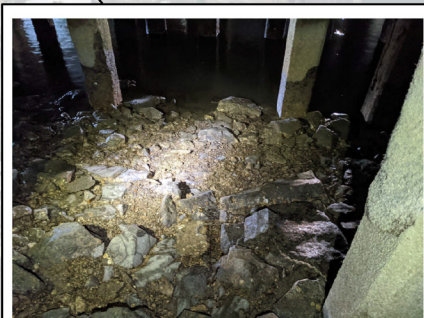
PHOTO 120 (P39_N_119117.jpg) Approxim a tely 75 ft 2 of exposed fill.
