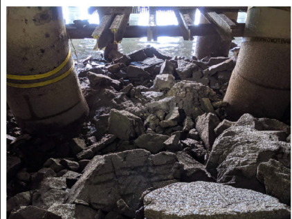
PHOTO 100 (P41_N_111112.jpg) Approxim a tely 50 ft 2 of revetm ent la cking la rge rock.
