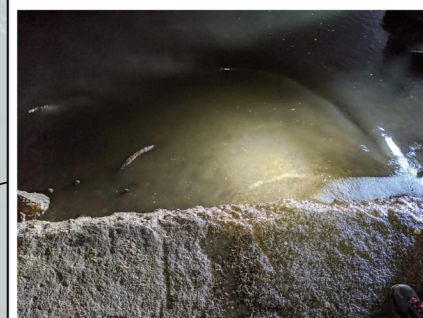
PHOTO 140 (CSD_N_2.jpg) Com bined Sewer Outfa ll invert, from a bove.
