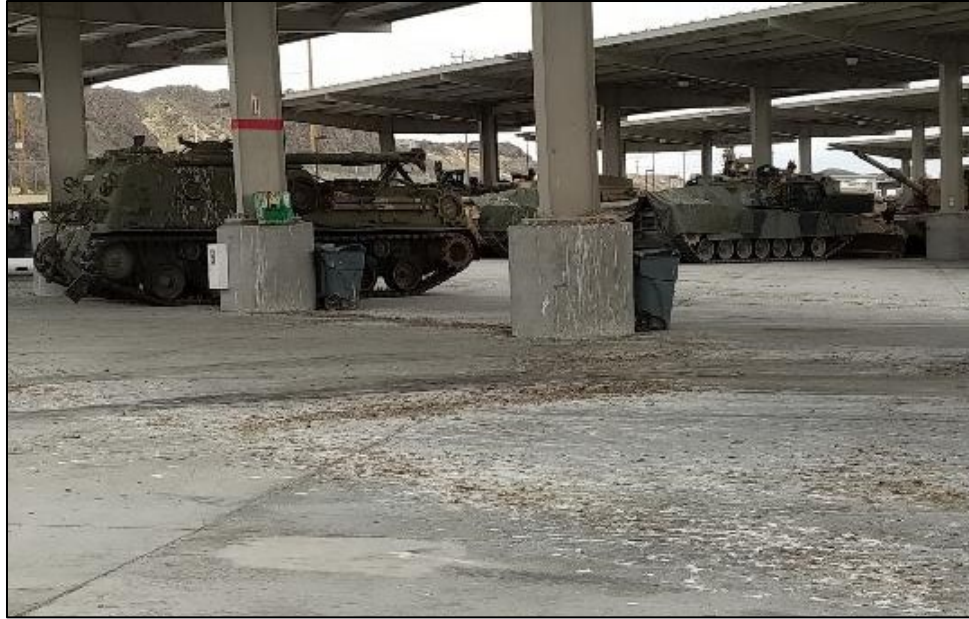
Photo 10 Raven Excreta after Installing Anti-Perching Devices at the 1 st Tanks Battalion yard at the Combat Center
