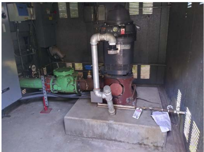
Left: Interior of pump enclosure, depicting the well seal, pipeline, and pump motor. Right: Overview of the subject property with the electrical service box at the right side of the frame. View to the south from the rear of the property.
