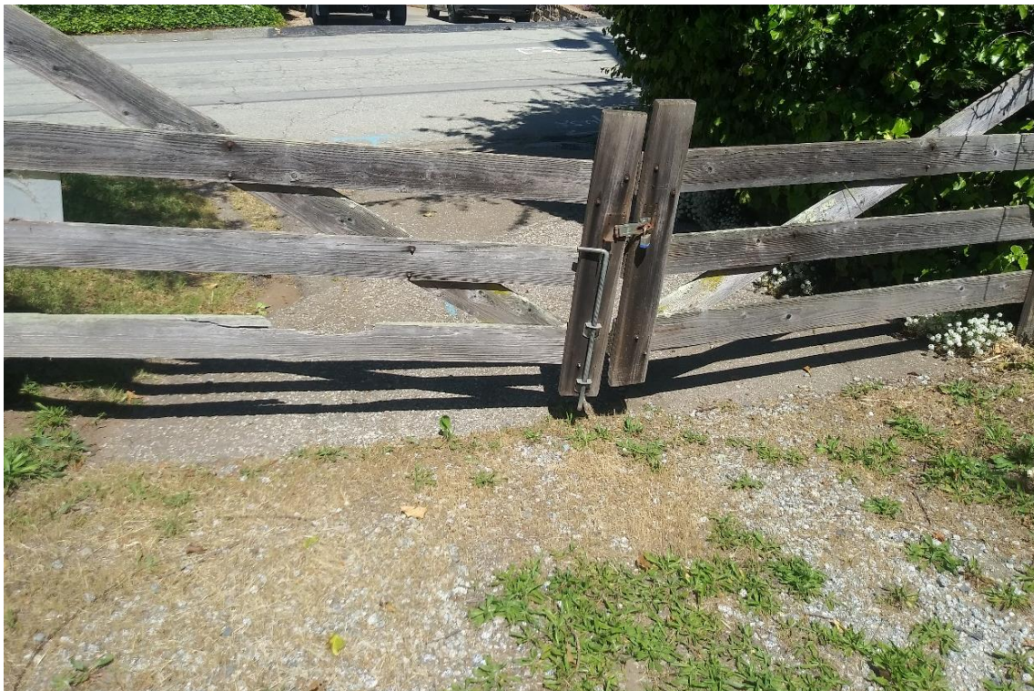
Figure 4 Gravel Driveway and Fence/Gate of Northwest Corner of Project Site
