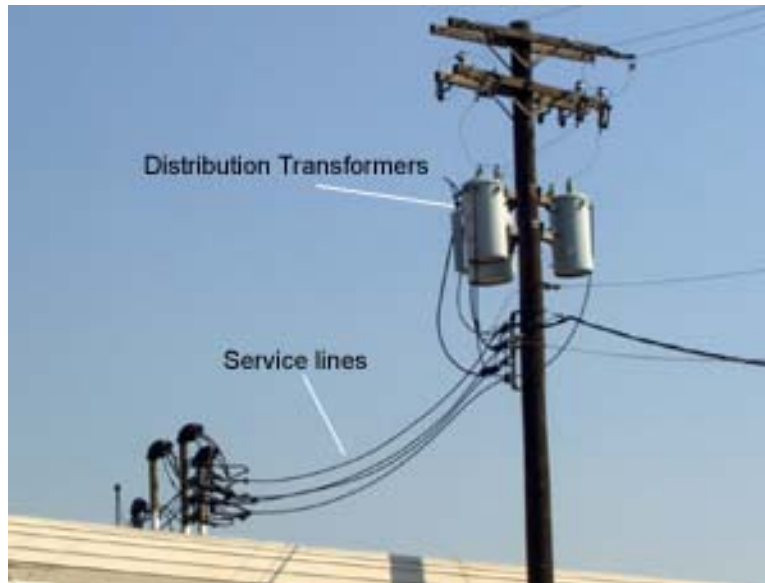
FIGURE 6: PROTOTYPICAL DISTRIBUTION CONNECTION
