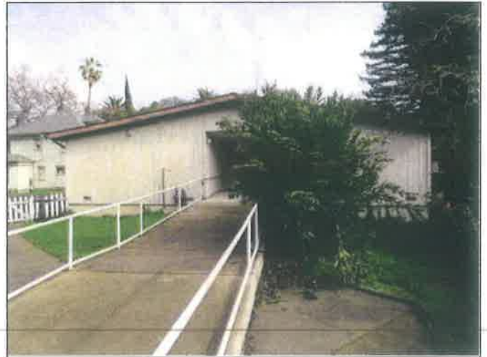
36. West side of the convalescent building
