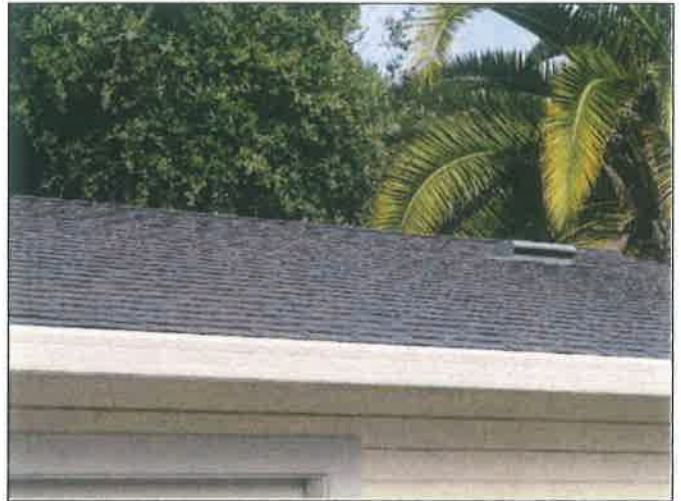
64. Composition shingle roofing at the garage building
