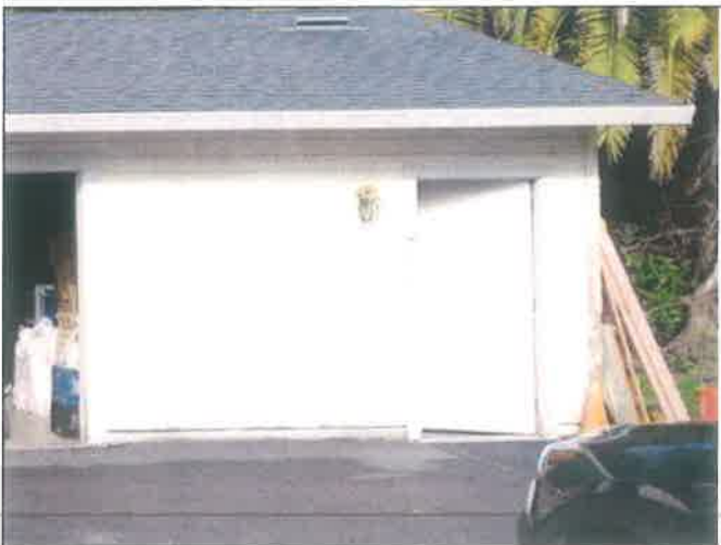
59. Entry door at the garage building
