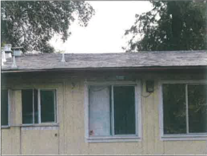
51. Windows at the convalescent hospital building
