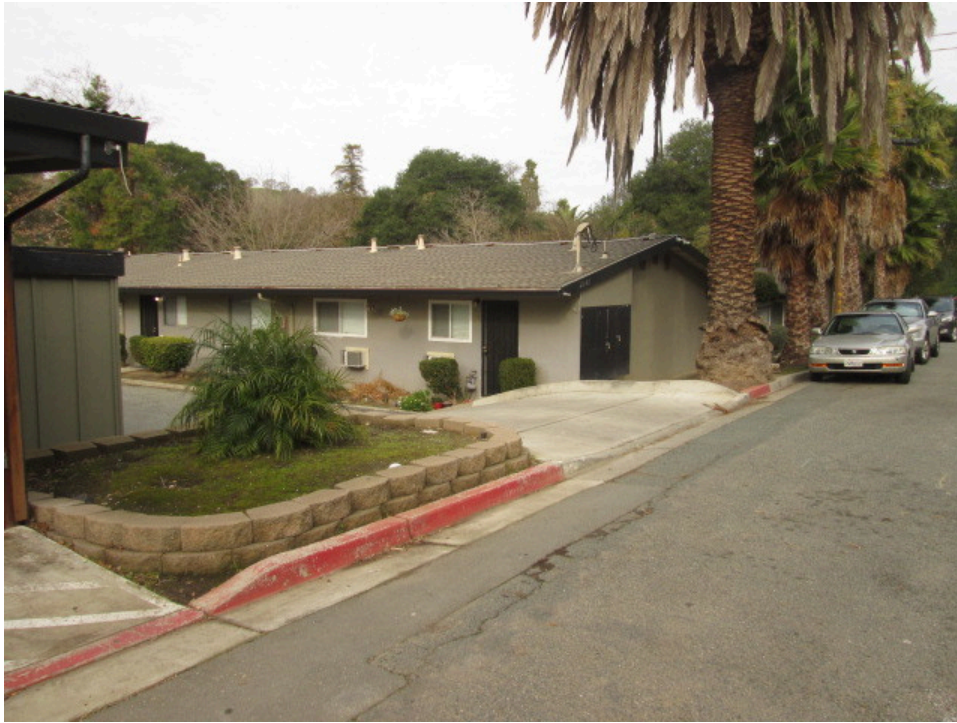
47. Apartments on the property to the north beyond the vacant lot
