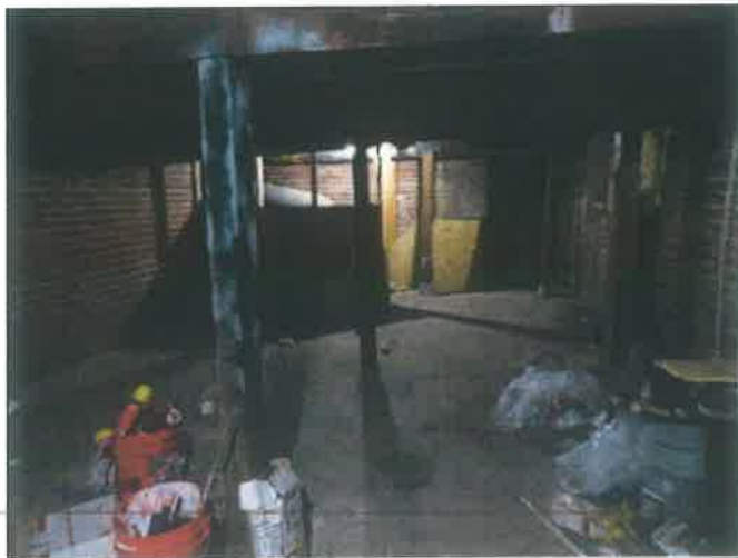
29. Concrete slab-on-grade at the residential building
