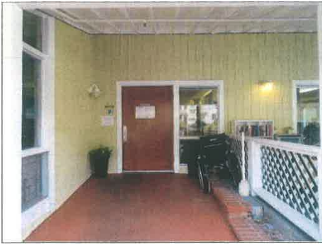
55. Main building entrance door and windows at the convalescent hospital building
