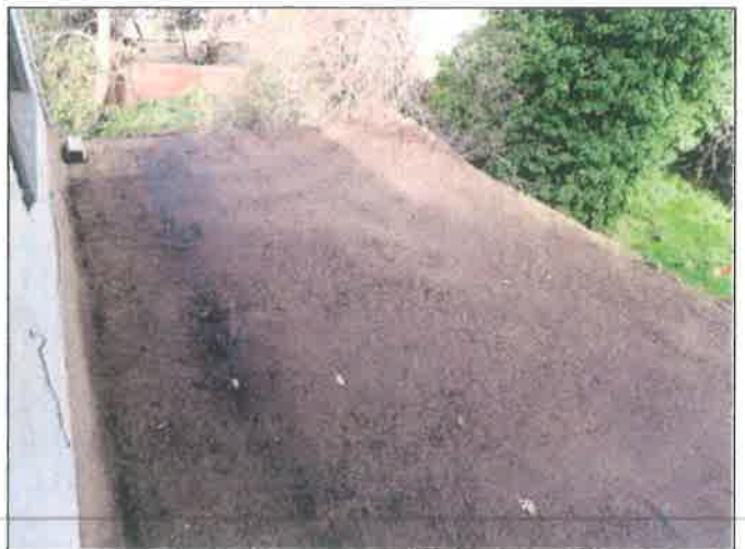
66. Porch canopy roofing BUR membrane
