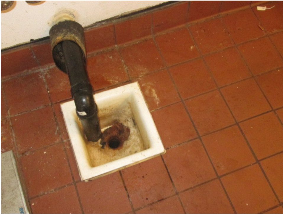
15. Floor drain in the kitchen
