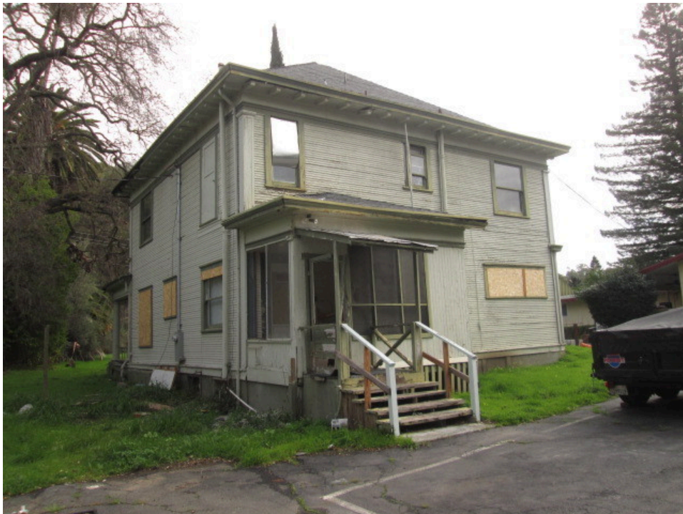
28. View of the house looking southeast
