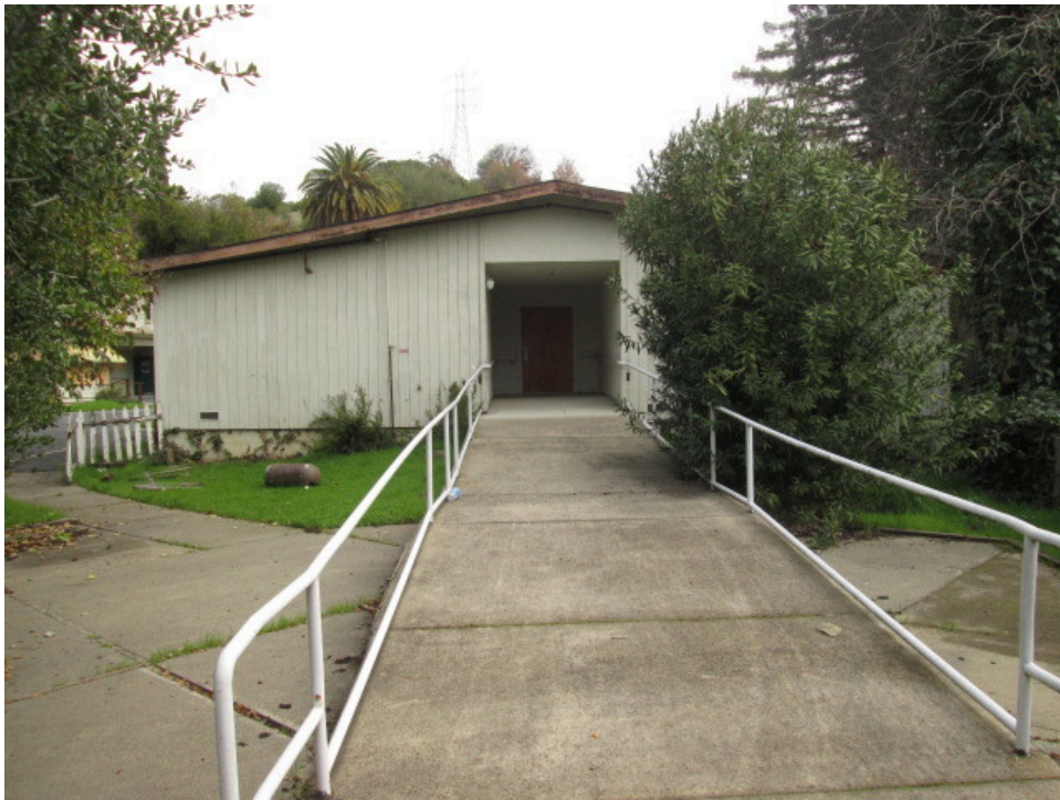
8. West facing side of the convalescent home
