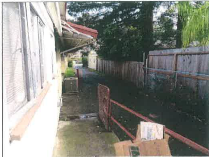
39. Southwest side of the building
