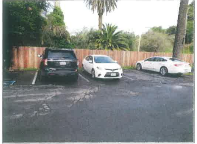
8. East parking area and parking stalls
