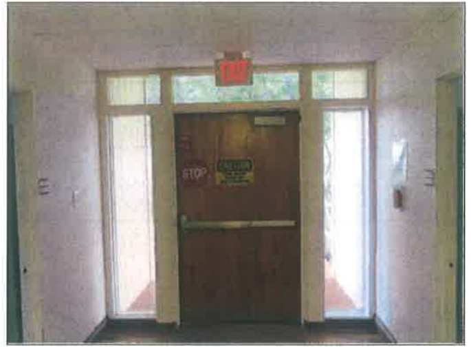
56. West building entrance door and windows
