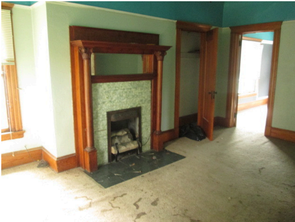
32. Second floor of the house
