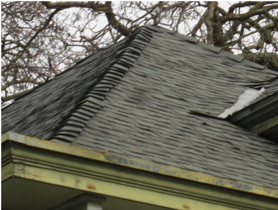
40. Roof of the house
