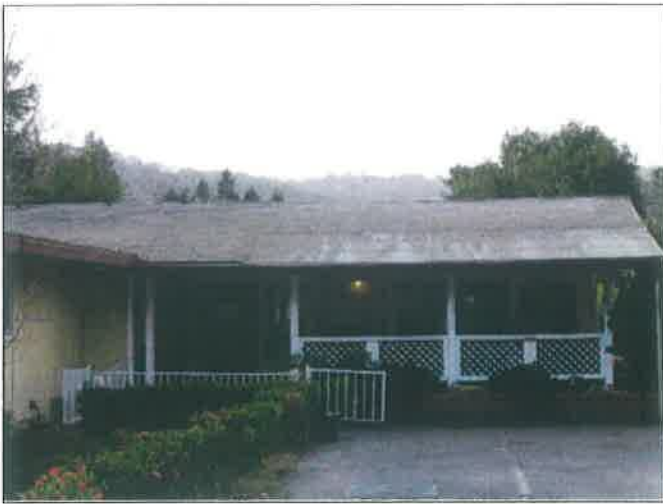
61. East portion of the convalescent hospital building roof
