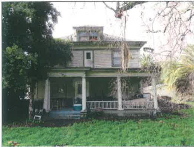
45. East side of the residential building
