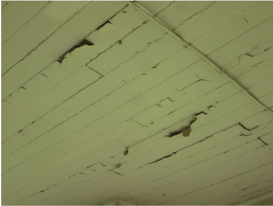
39. Flaking exterior paint at the house
