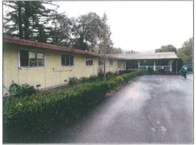
34. Northeast portion of the convalescent hospital building
