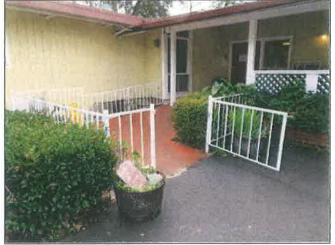
10. Entrance walkway at the convalescent hospital building. Note landscaping.
