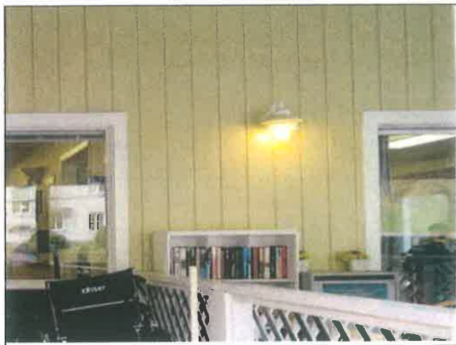
21. Building-mounted light fixture at the convalescent hospital building
