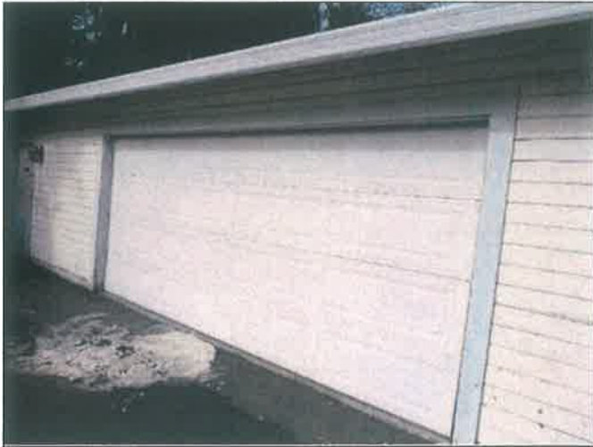
57. Overhead door at the garage building
