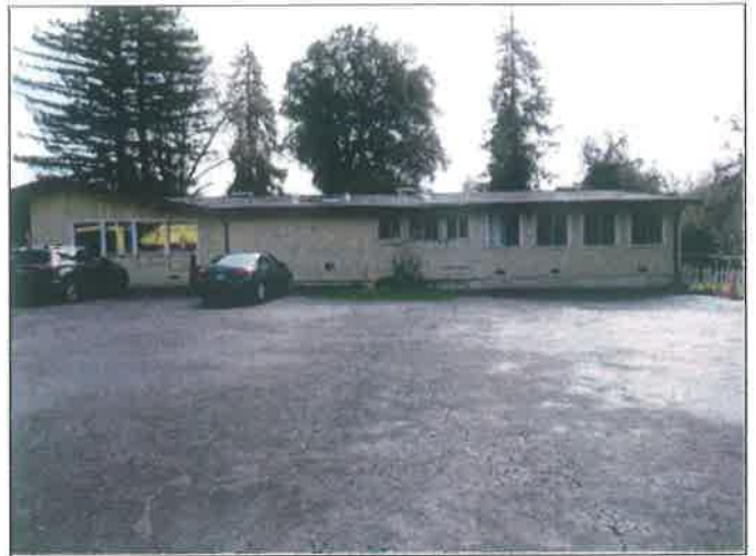
38. Northwest portion of the convalescent building
