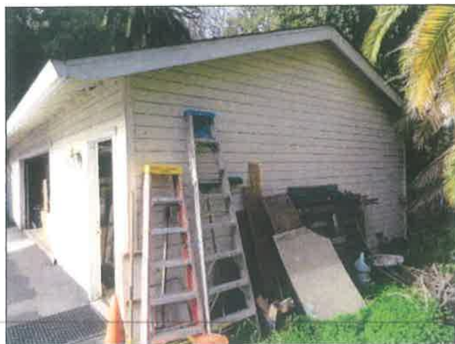
41. East side of the garage building
