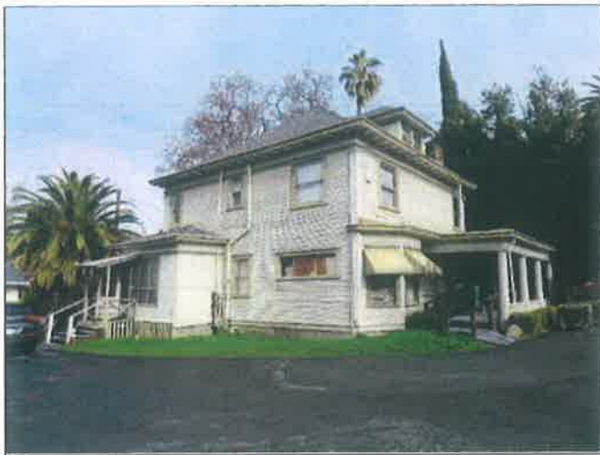
43. West and south sides of the residential building
