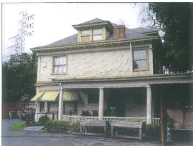
47. South side of the residential building showing porch framing
