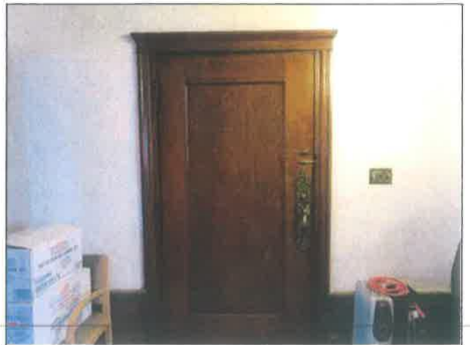
60. Main entry door at the residential building
