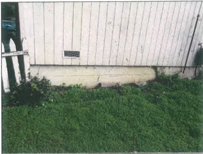
27. Perimeter strip foundation at the convalescent hospital building
