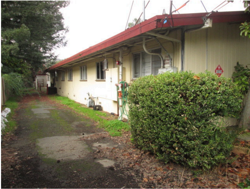
7. South facing side of the convalescent home
