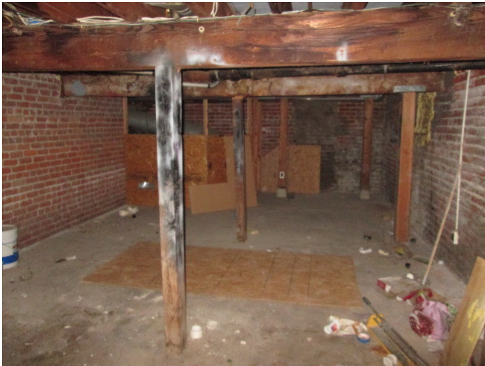
34. Basement of the house
