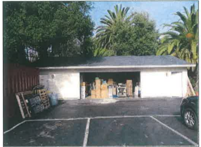
40. South side of the parking garage building
