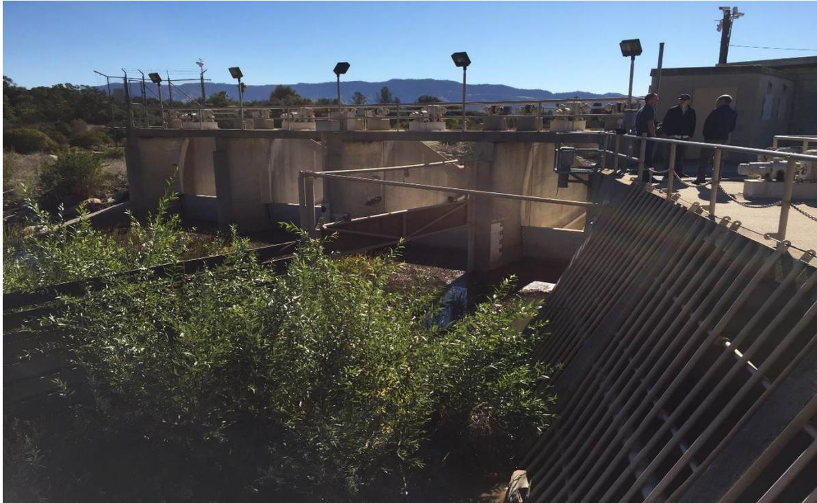
**Photograph 7.** View of upstream side of the spillway, radial gates and headworks (December 13, 2019).
