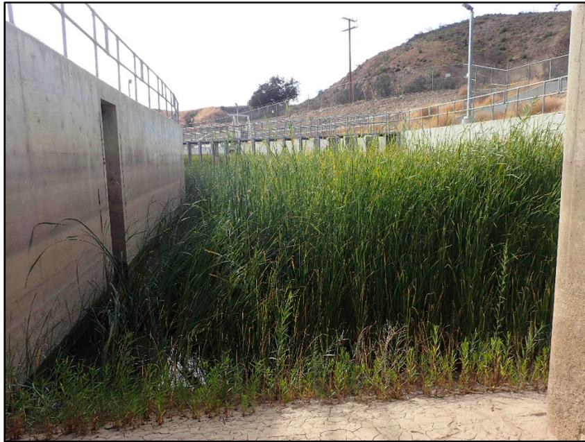
**Photo 11- Dense vegetation and sediment deposition in Robles Diversion screenbay**
