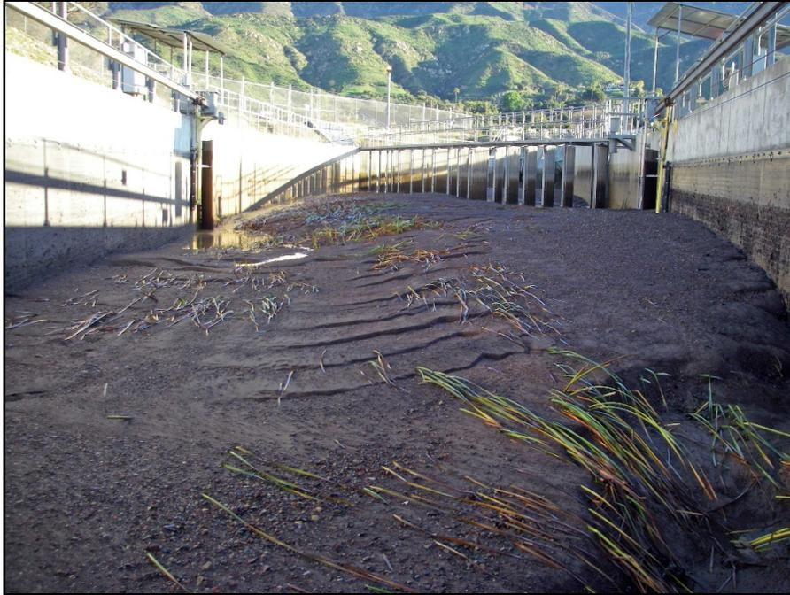
**Photo 13- Sediment inundation in Robles Diversion screenbay prior to emergency cleanout**
