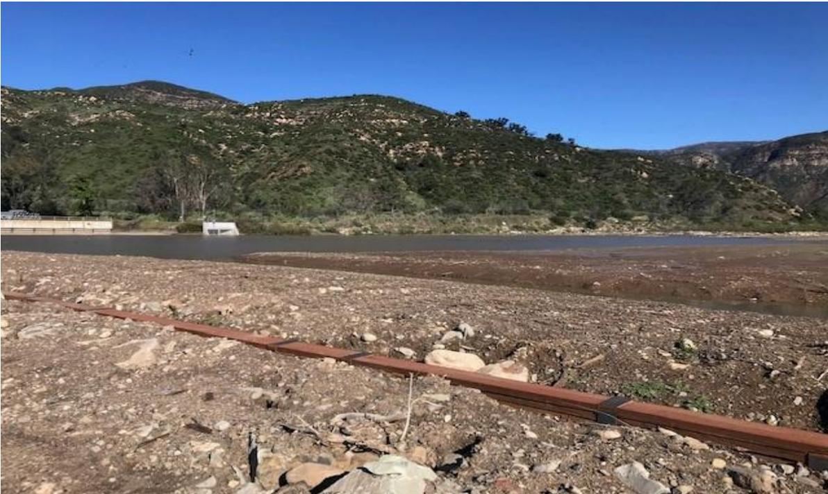
**Photograph 2.** View of the timber cut-off wall after repairs to the wall were made in November 2019. Light vehicles can drive over the timber cut-off wall to access the fish passage facility to the west, without driving through the active flowing channel (February 2, 2020).
