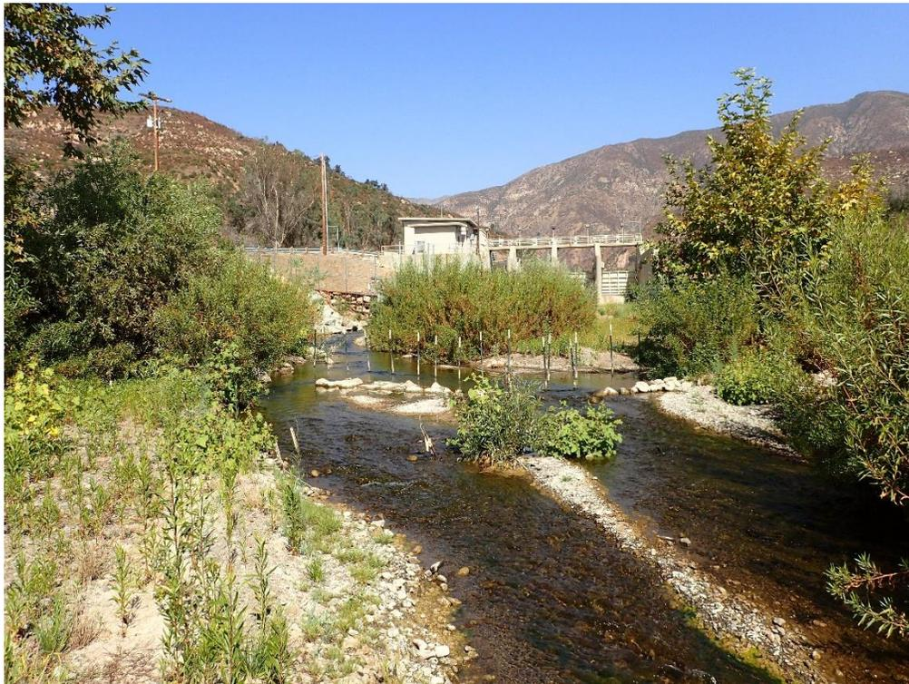
**Photograph 6.** Sediment deposition downstream of Robles Diversion
