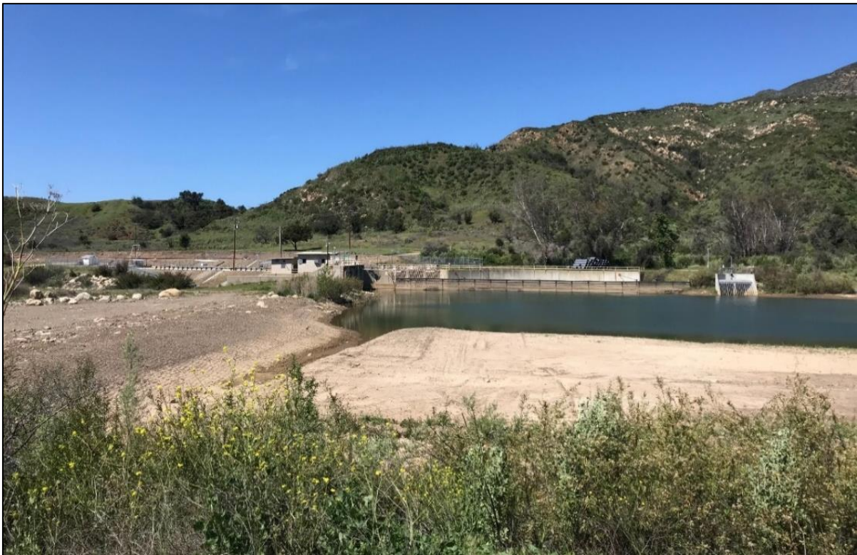
Figure 15 Overview of the Robles Diversion Dam Facility, View West
