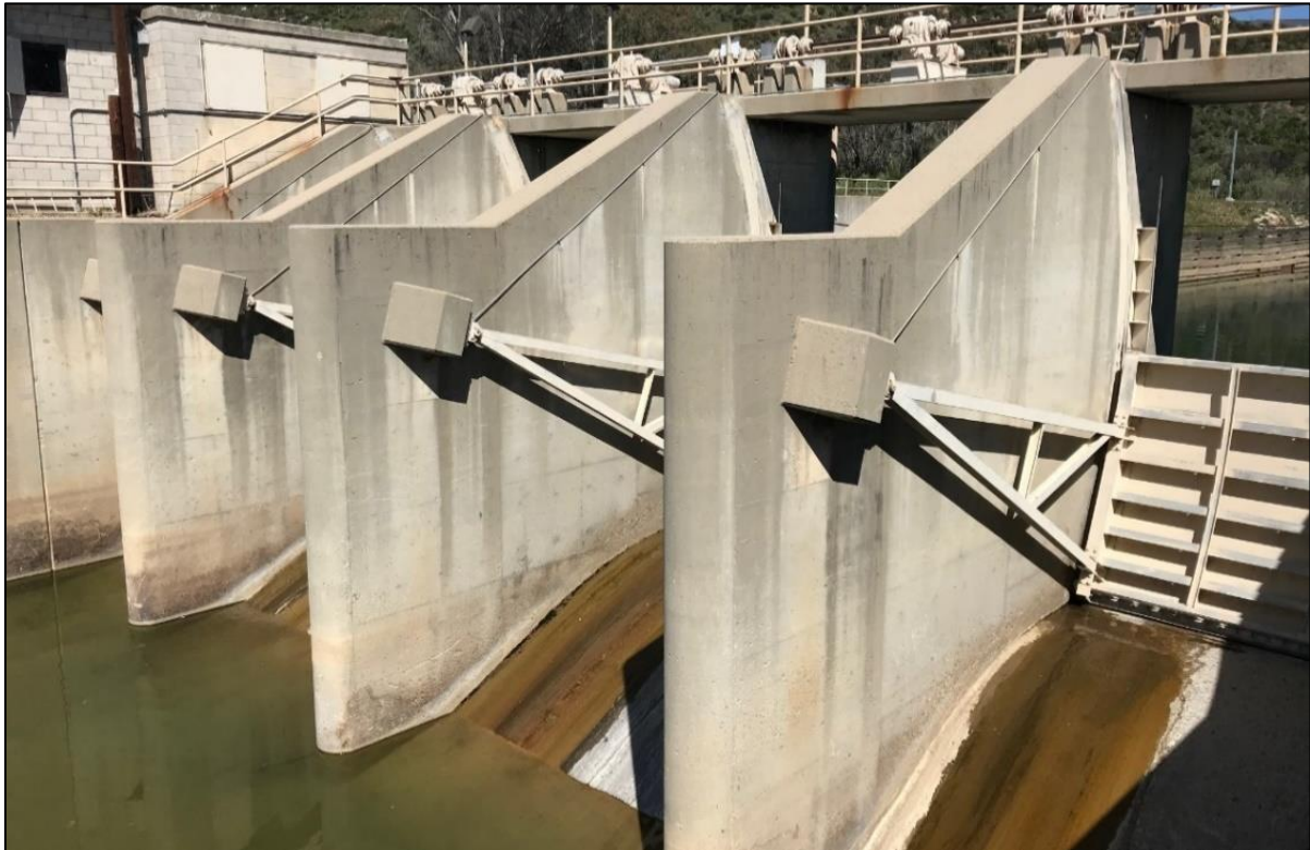
Figure 16 Robles Diversion Dam Gates View North
