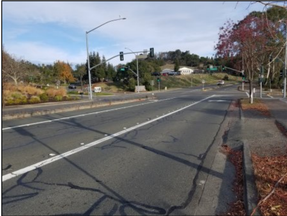
14 : View down Fountaingrove Parkway, facing north.
