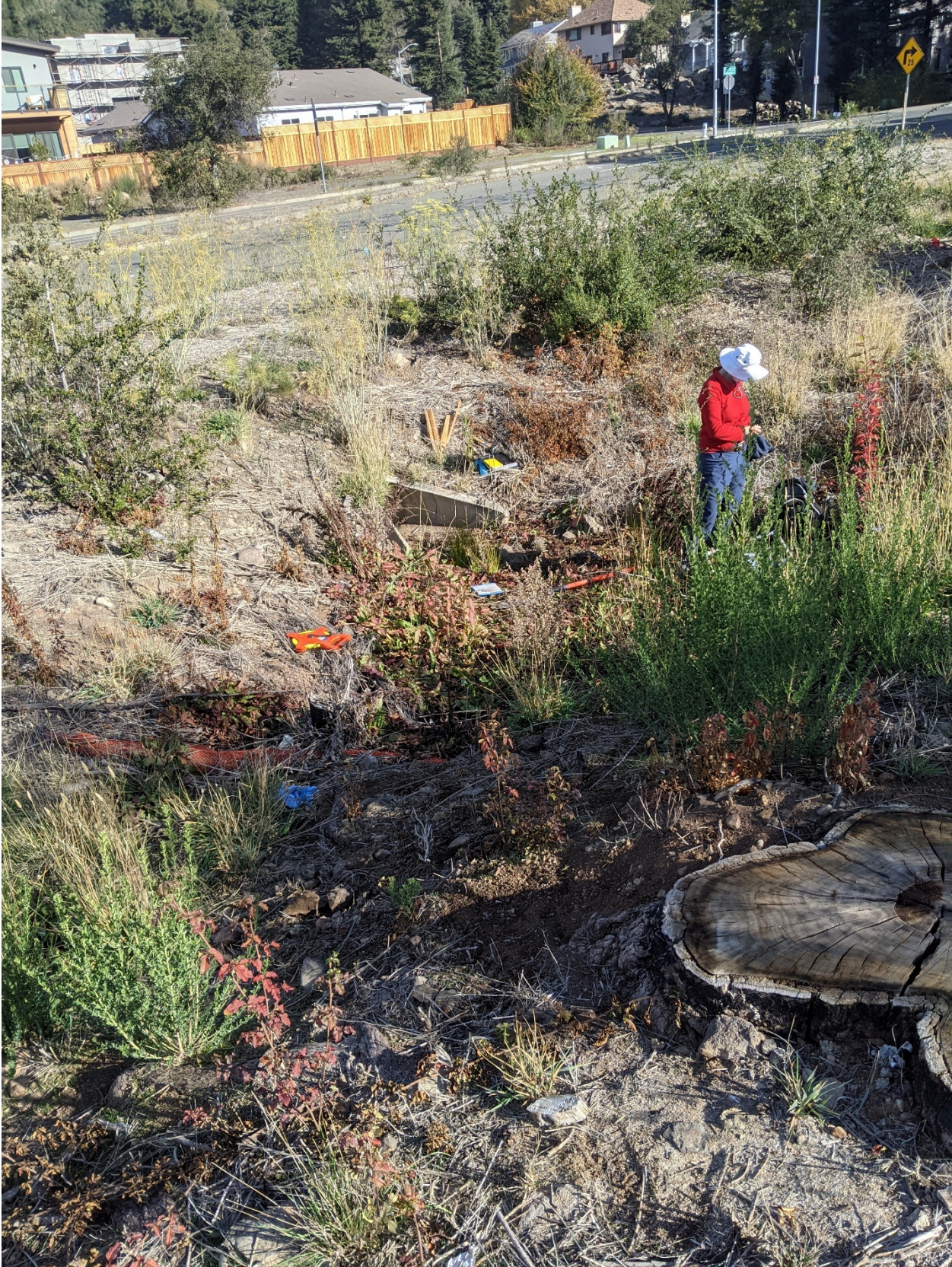
Photo 5: Cross Section 1 at storm drain outlet.
