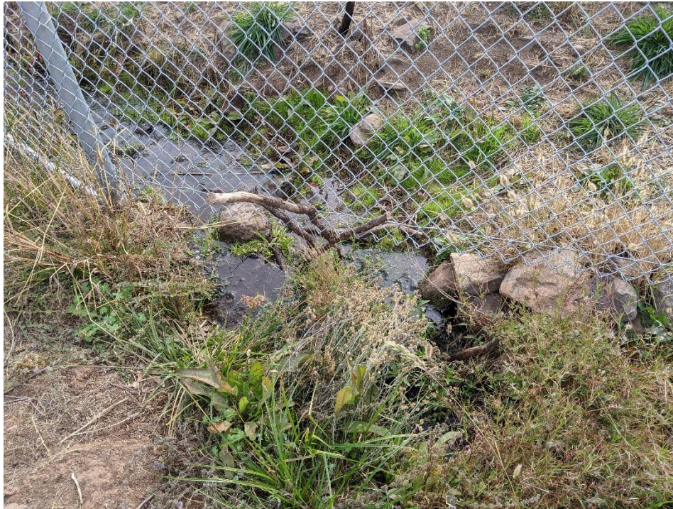
Photo 4. A view of inundation within the potentially jurisdictional perennial drainage, along the fenceline bordering the southern portion of the project site. Taken November 11, 2020.
