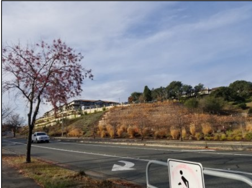
16 : View of the Varena Design Center retirement home, to the west of the site.
