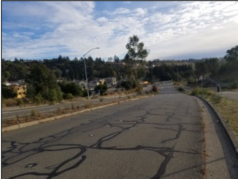
10 : View down Stagecoach Road, facing east.
