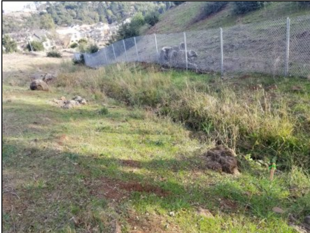
6 : View of the drainage ditch on the central portion of the site.
