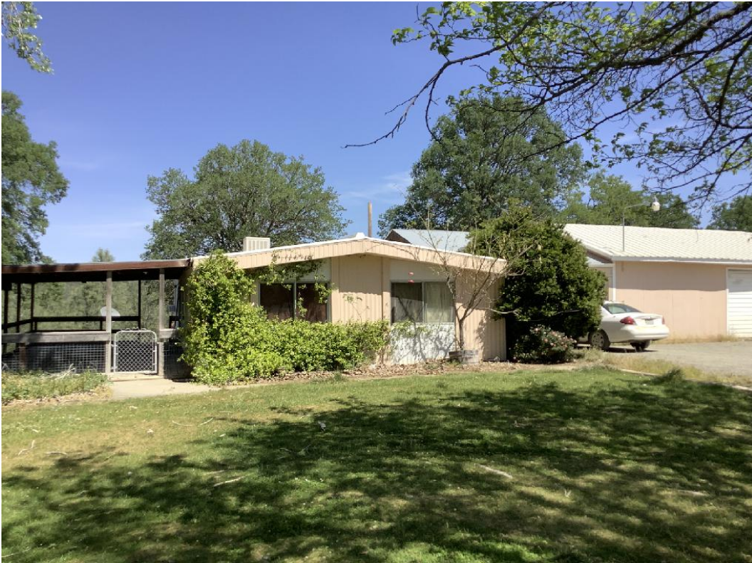
Photo 1: Residential Structure within Study Area 1 is proposed to be converted to an indoor nursery.
