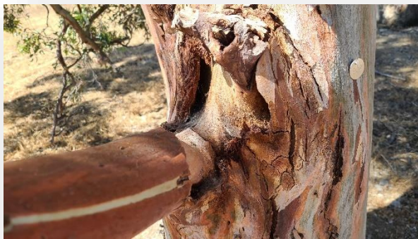
Plate 2. This a view of a cavity with internal decay above a branch collar (#902).
