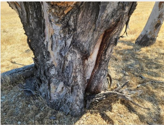
Plate 14. This is a view of a decay at a stem flare (#924).
