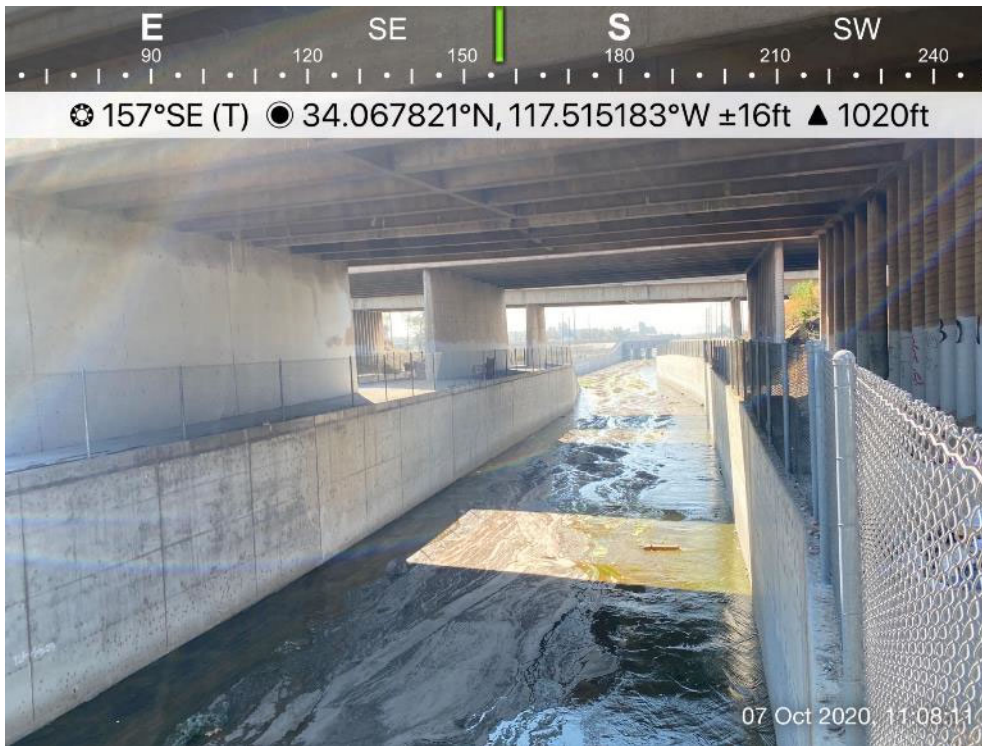
Photo 5. View of concrete drainage downstream
