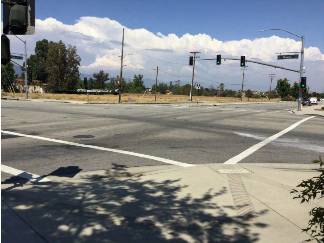
Figure 5-9. Overview of segment of Baseline Road that intersects the Project and Etiwanda Avenue from the southwest corner of the intersection, facing northeast
