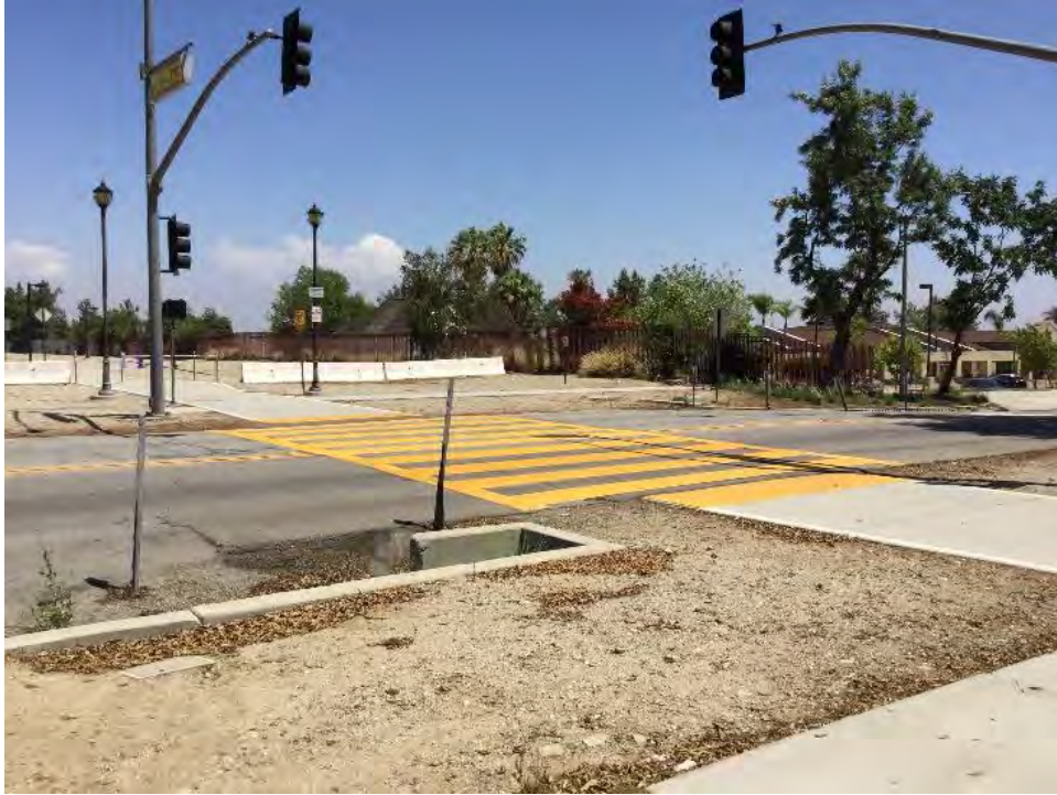
Figure 5-10. Overview of segment of former Pacific Electric Line at Etiwanda Avenue; rail line has been demolished and converted to a walking/bike path, facing southeast
