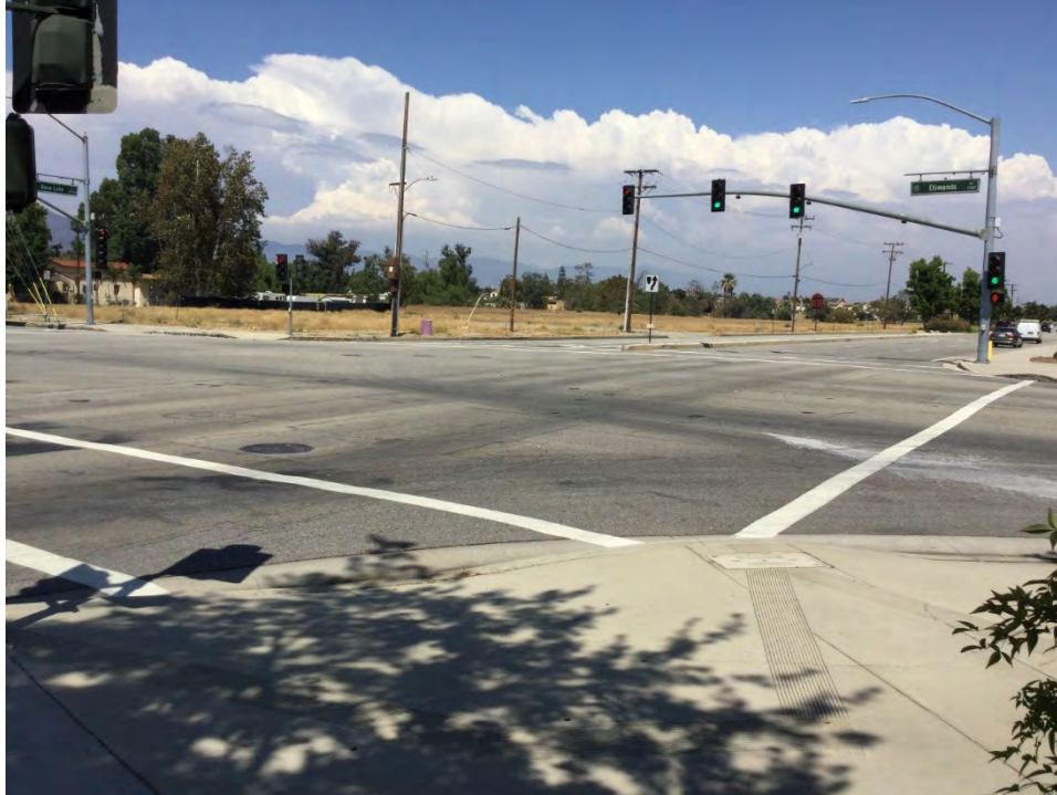
Photo: Overview of segment of Baseline Road that intersects the Project and Etiwanda Avenue from the SW corner of the intersection, facing NE
