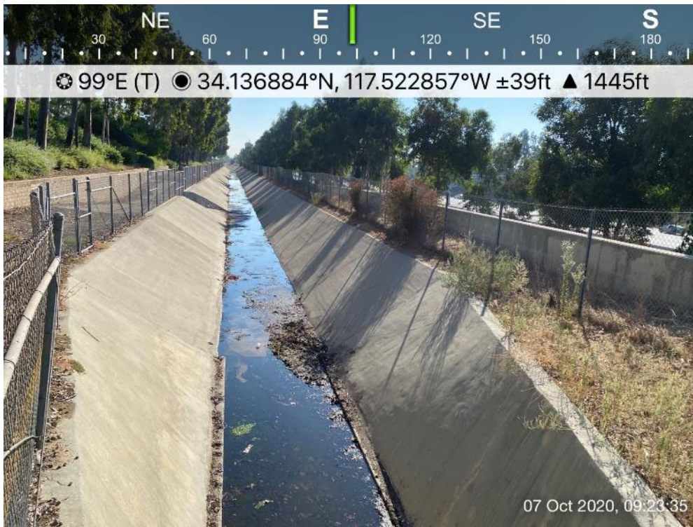
Photo 1. View of unnamed Drainage looking east (upstream) north of SR 210.
