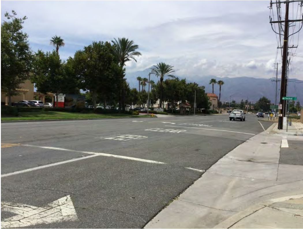
Figure 5-6. Overview of southern end of location of 36-007099 along Etiwanda Avenue, facing northwest.
