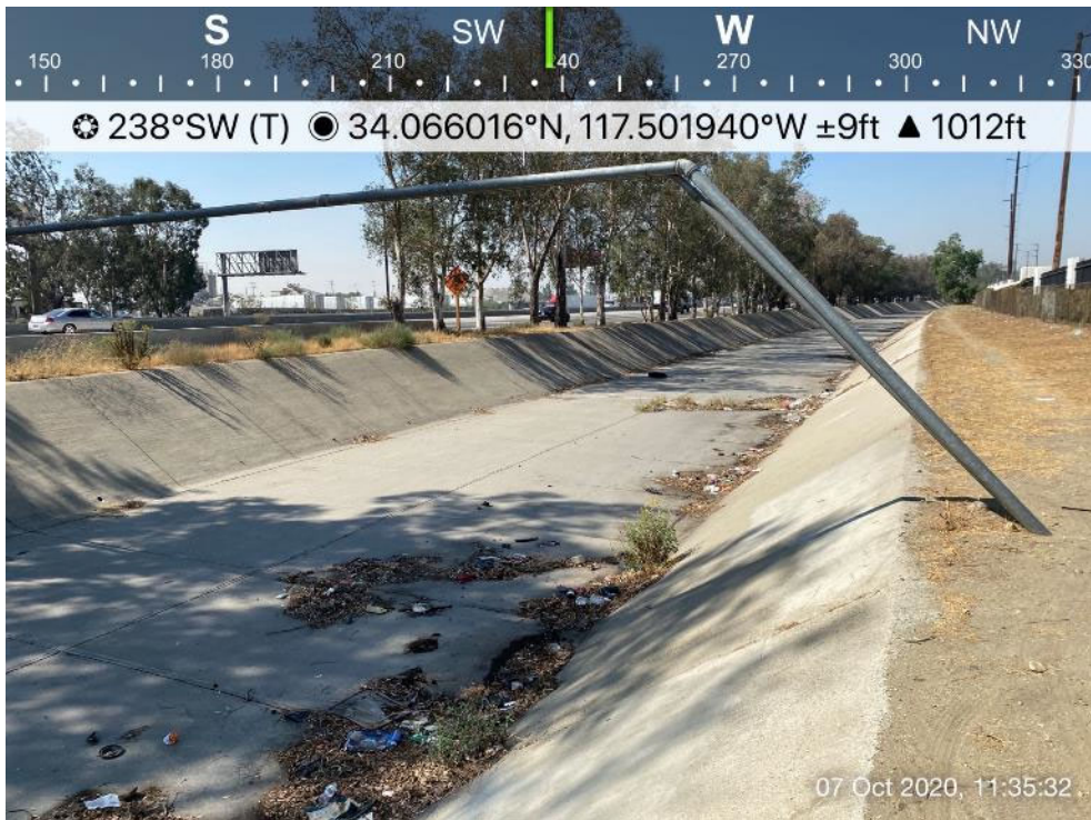
Photo 7. Looking southwest (upstream) at Caltrans flood control Drainage north of I-10.
