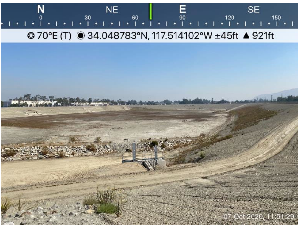
Photo 8. Looking northeast showing large flood control basin north of Jurupa Avenue.
