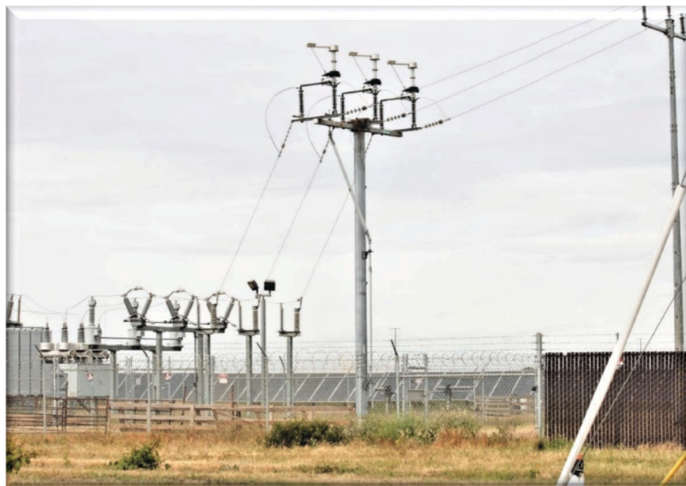
Plate 4. Swainson's hawk nest in the Kammerer substation, 2021.
