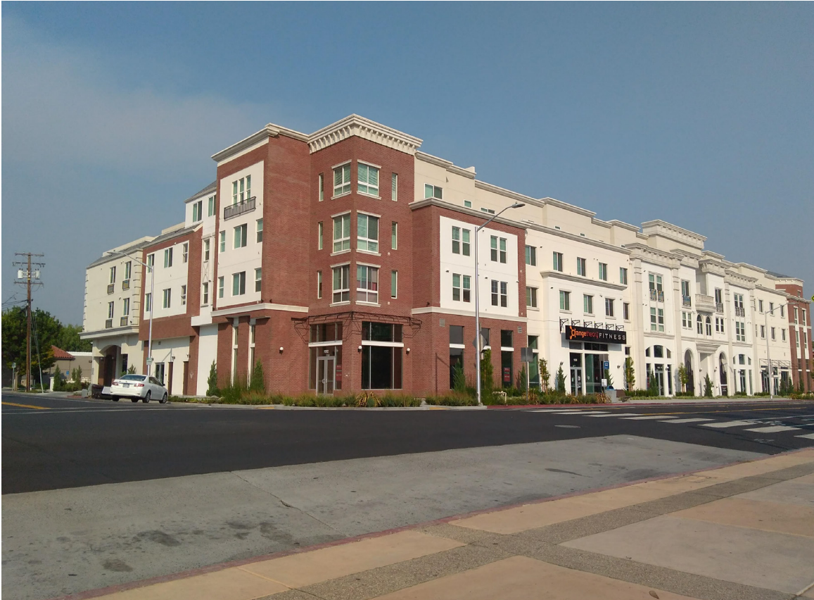
Photo 3: Views of mixed use commercial building north of the project site.
