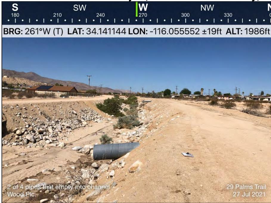
**Photo 9.** Photo showing two of the four corrugated steel culvert outlets that drain urban runoff into the channel.
