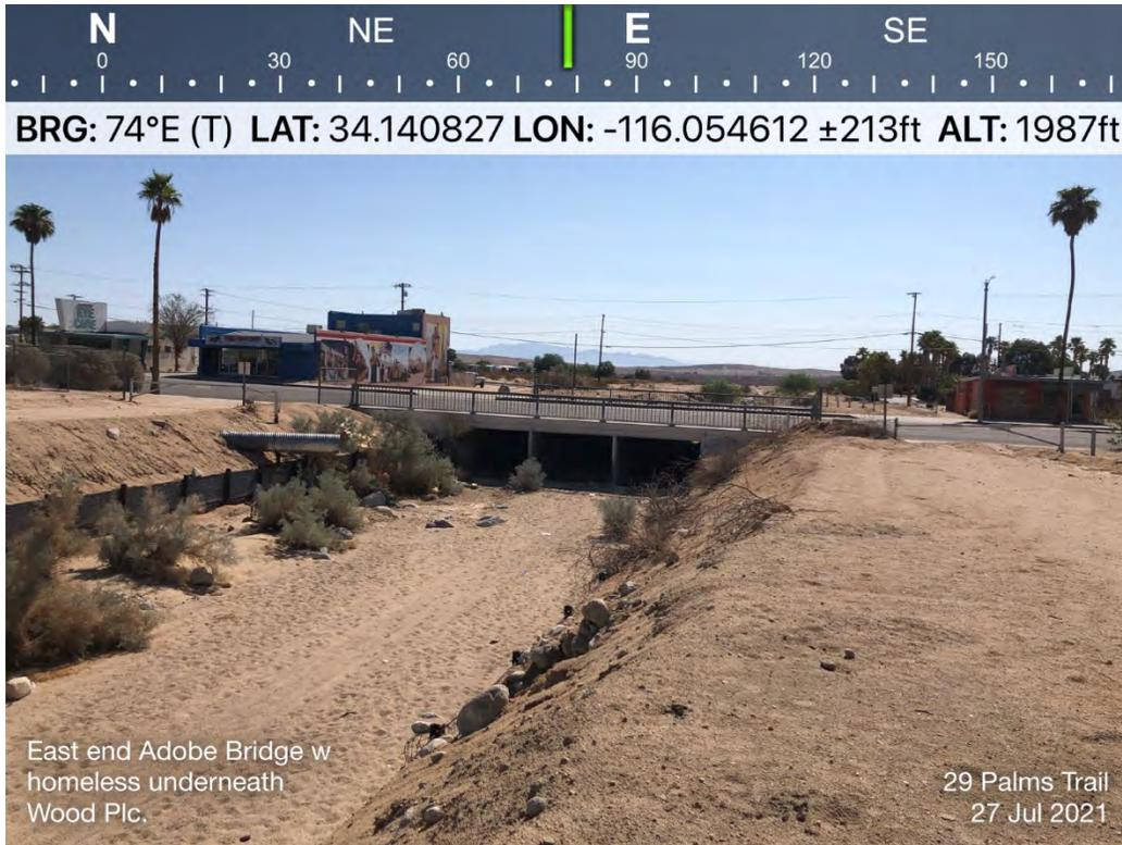
Photo 5. Looking east (downstream) showing the box culvert crossing at the Adobe bridge.
