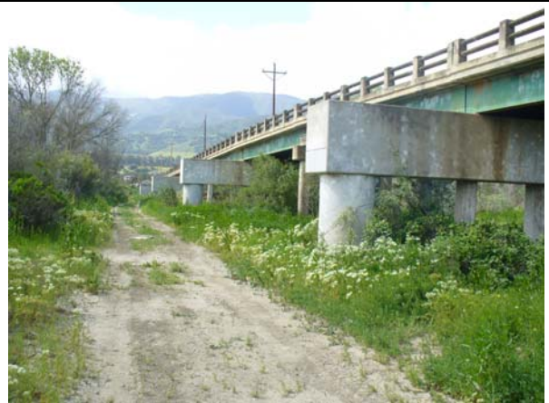
Photo 6: View of southern bridge structure from Salinas River bed looking south.
