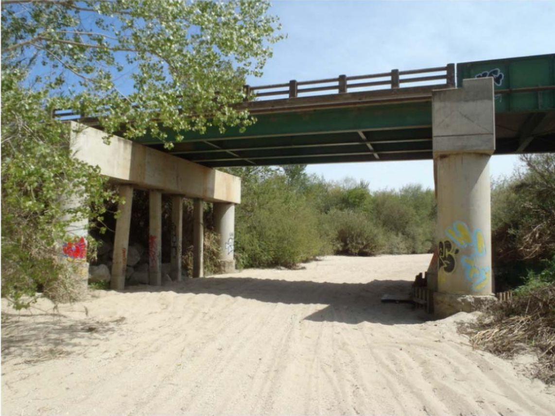
Photo 2. River Channel within Span 28 (Looking East)
