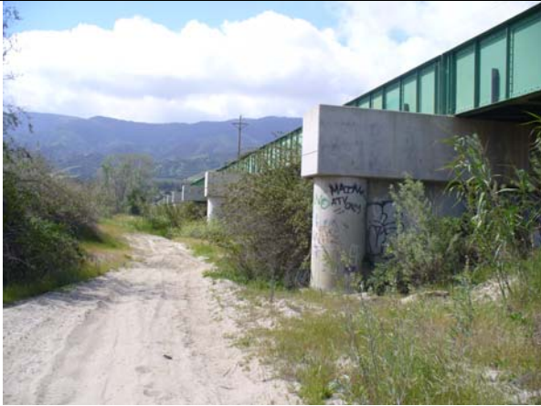
Photo 3: View of bridge structure from Salinas River bed looking south.
