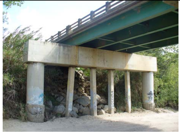
Photo 2: View of northern bridge substructure and abutment.
