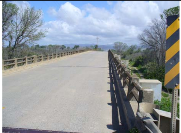
Photo 10: View of southern bridge roadway and guard rails.
