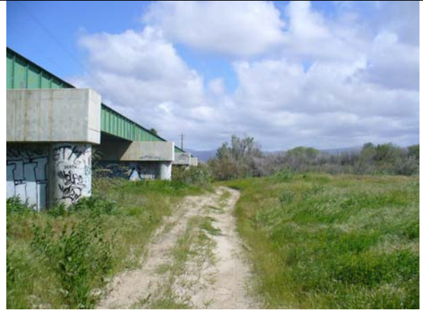
Photo 4: View of bridge structure from Salinas River bed looking north.
