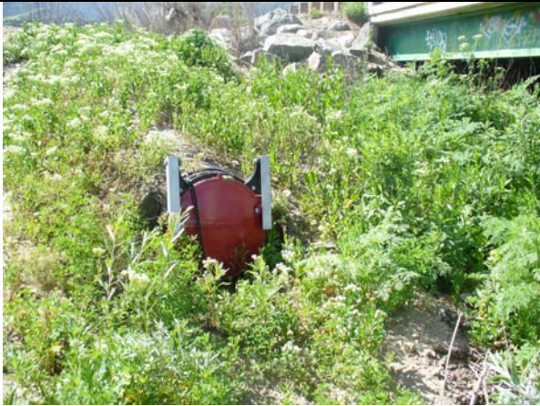
Photo 9: View of capped pipe near southeast corner of southern bridge terminus.
