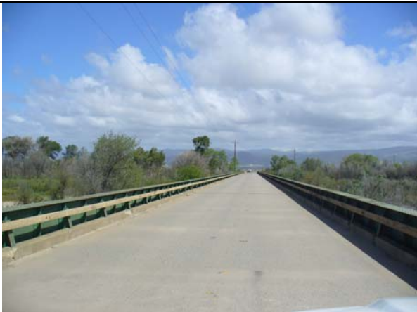
Photo 11: View of northern bridge roadway and guardrails.
