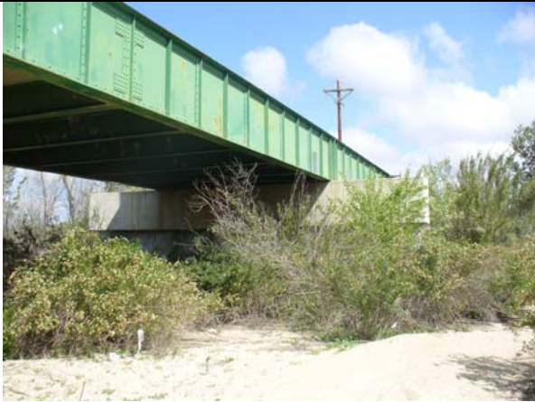
Photo 1: View of bridge substructure from Salinas River bed, looking north.
