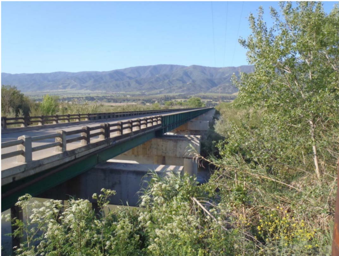
Photo 1. Existing Bridge (Looking West)
