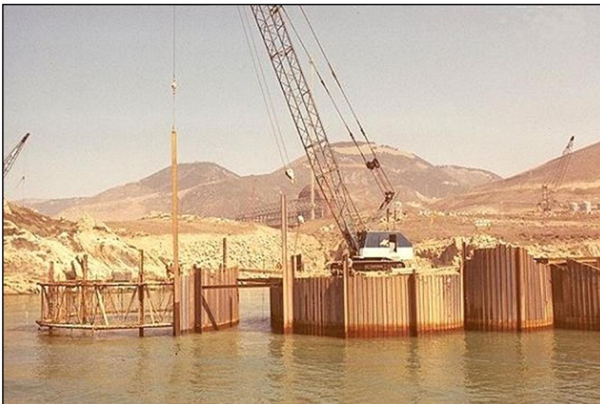
Source: PG&E, 2022c – Figure 4.1.1-3, Threading Sheets.
