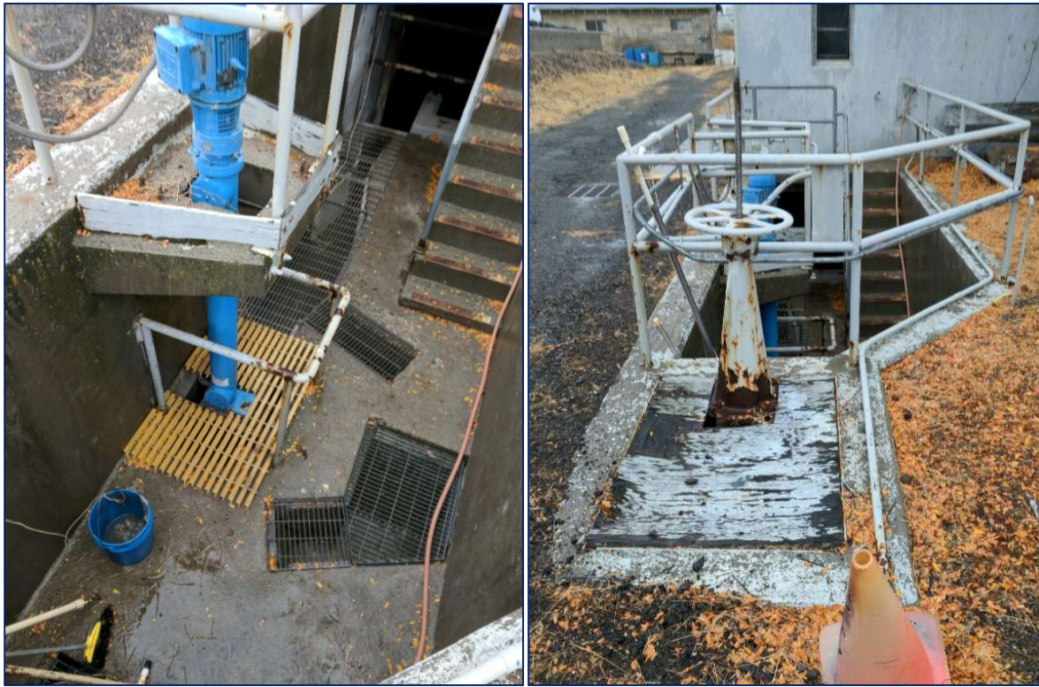
Figure 7. Grinder and bar screen bypass.
