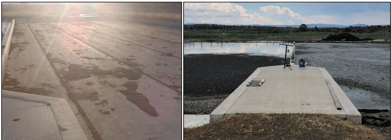
Figure 17. Sludge drying beds.
