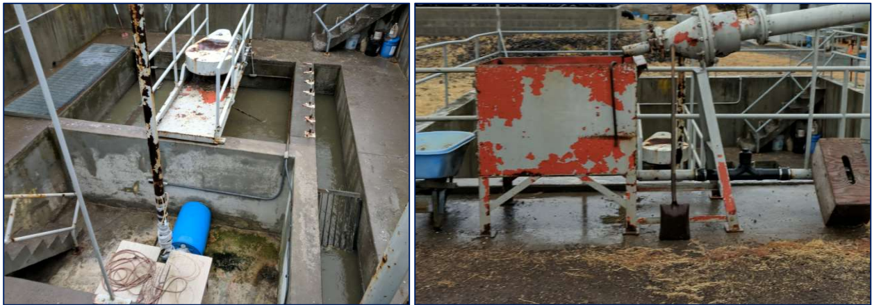
Figure 6. Existing bar screen and grit chamber
