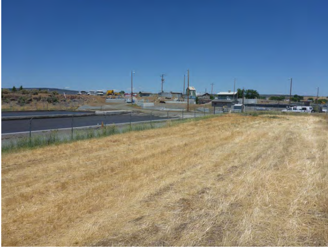
City of Alturas wastewater treatment plant
