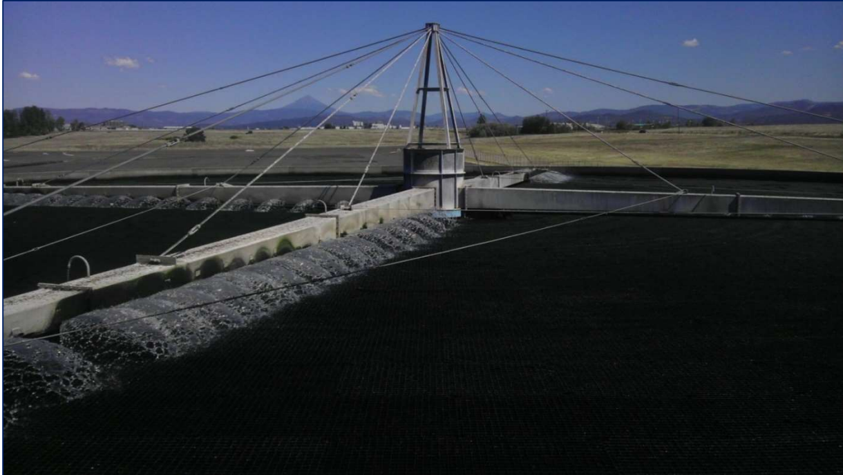
Figure 21. Typical trickling filter showing media as is recommended for Alturas.
