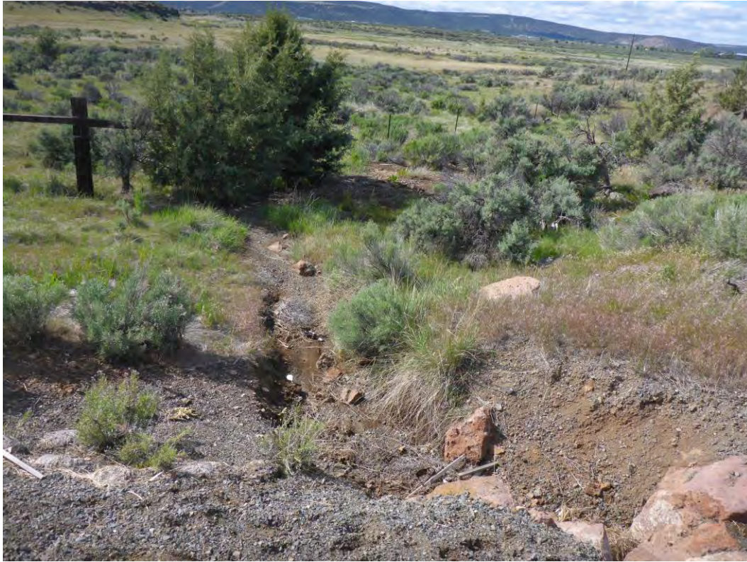
Non-jurisdictional erosional rill channeling roadside runoff to uplands, view to north. Midway between 8:WM and Westside Road (County Road 60).
