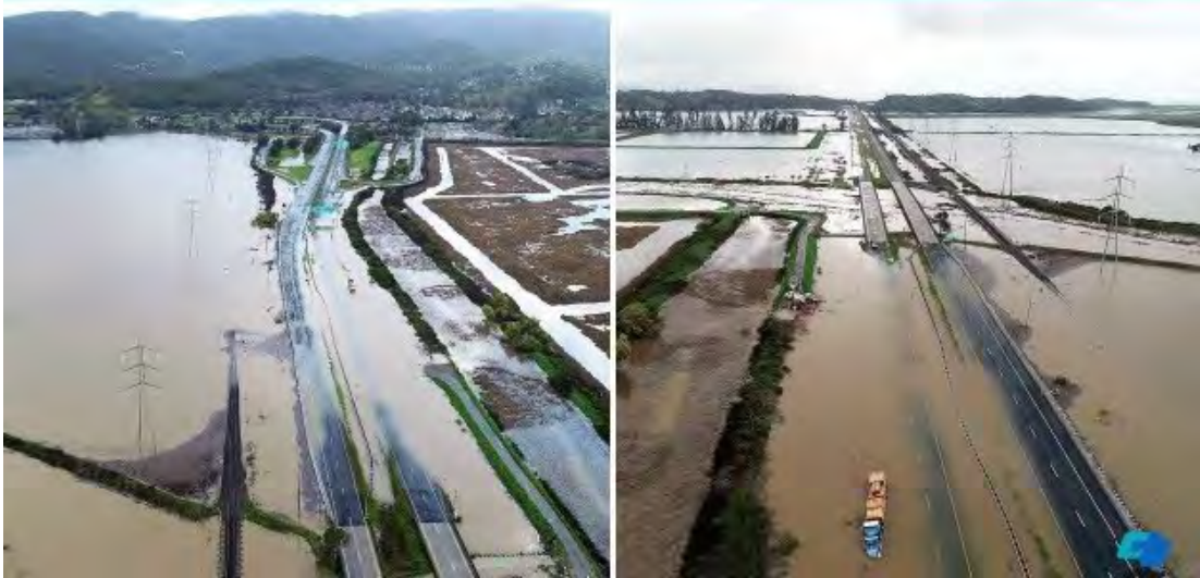
Photo 1. 2019 Flooding. Looking west on SR 37 at Novato Creek (left).
