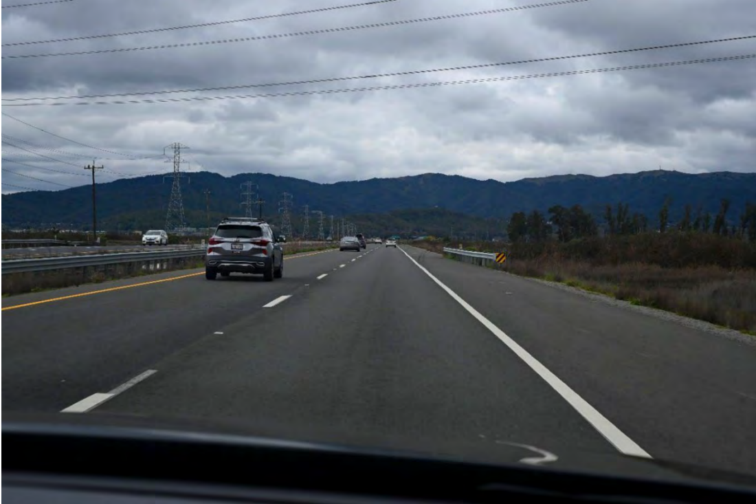
Figure 2.1.8-6. Existing Condition KV-2
