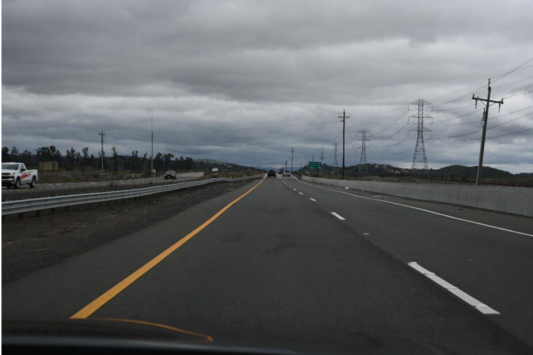
Figure 2.1.8-3. Existing Conditions KV-1
