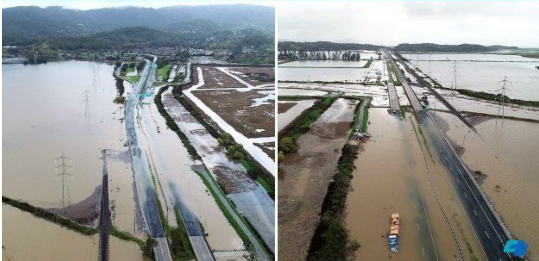
Photo 1. 2019 Flooding. Looking west on SR 37 at Novato Creek (left).
