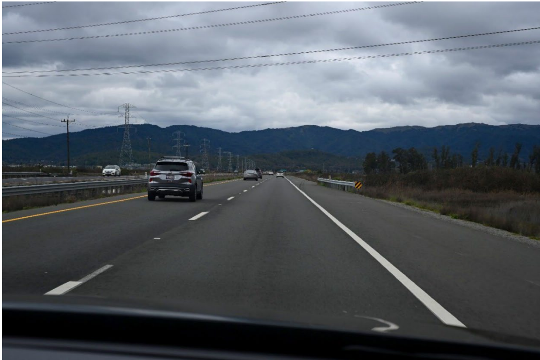
Figure 2.1.8-6. Existing Condition KV-2
