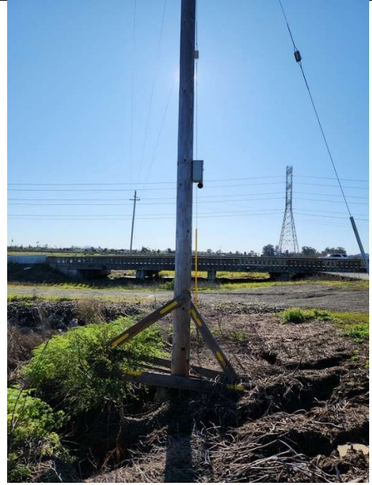
LT-2: Service Road to Marin County Flood Control and Water Conservation District
