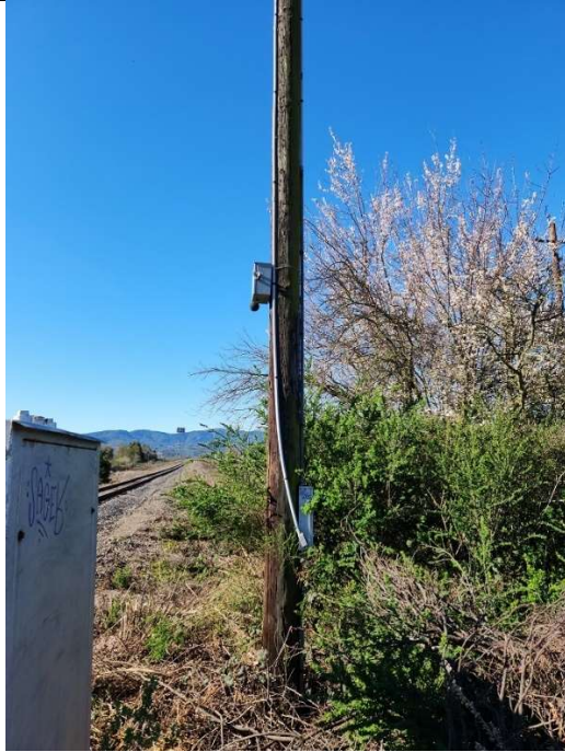
LT-1: Along train tracks near SR 37/Atherton Avenue intersection
