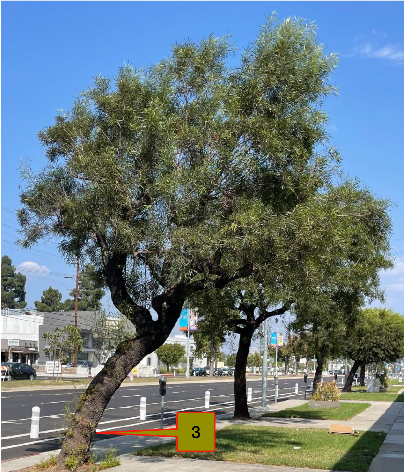
PHOTO - Shows City of Los Angeles street tree #3. Tree has a pronounced lean and an asymmetrical canopy. Trees #1 through #7 are recommended for removal and replacement.
