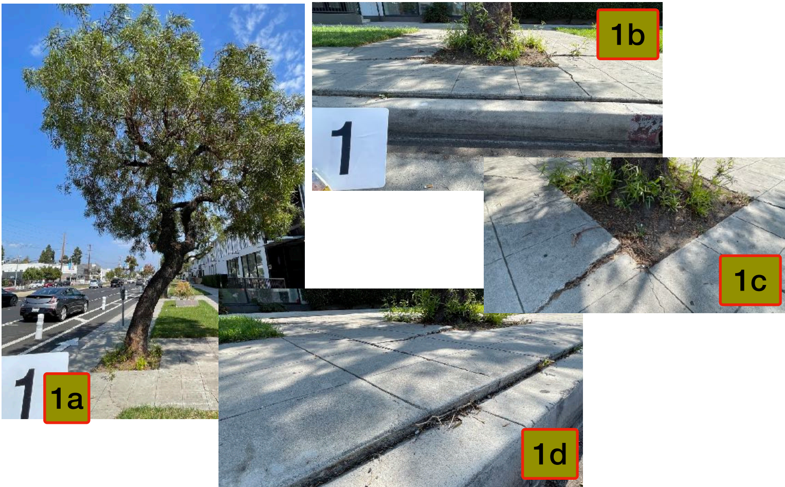
PHOTO 5 - Shows City of Los Angeles street tree #1, recommend for removal.
