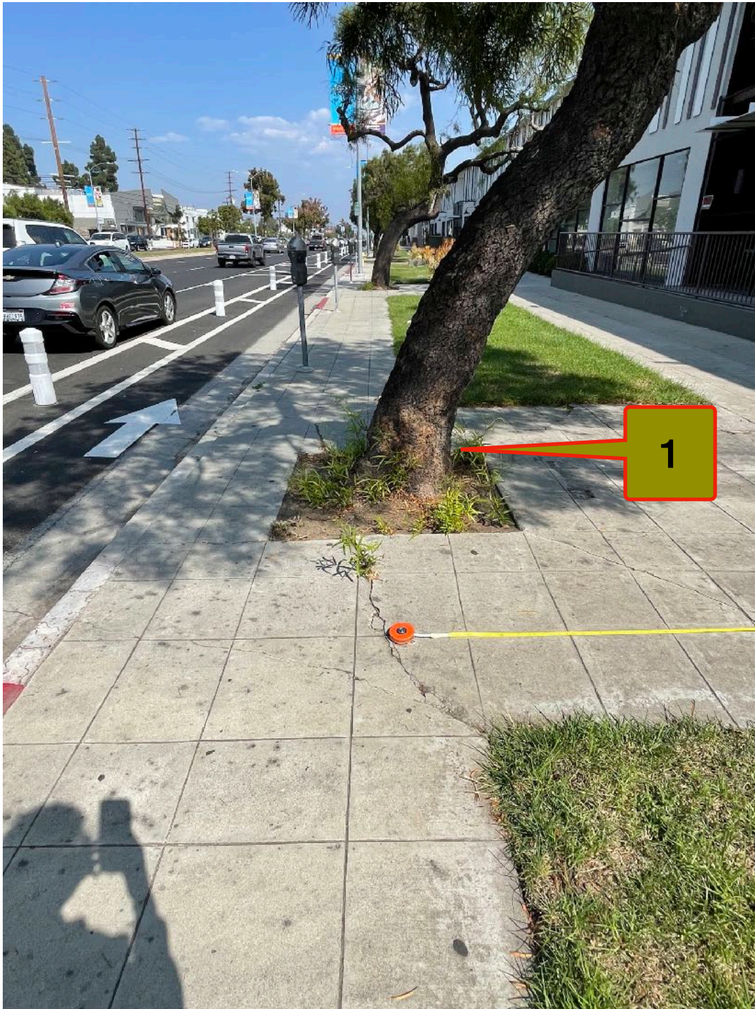
PHOTO 4 - Shows City of Los Angeles street tree #1 with prominent lean.
