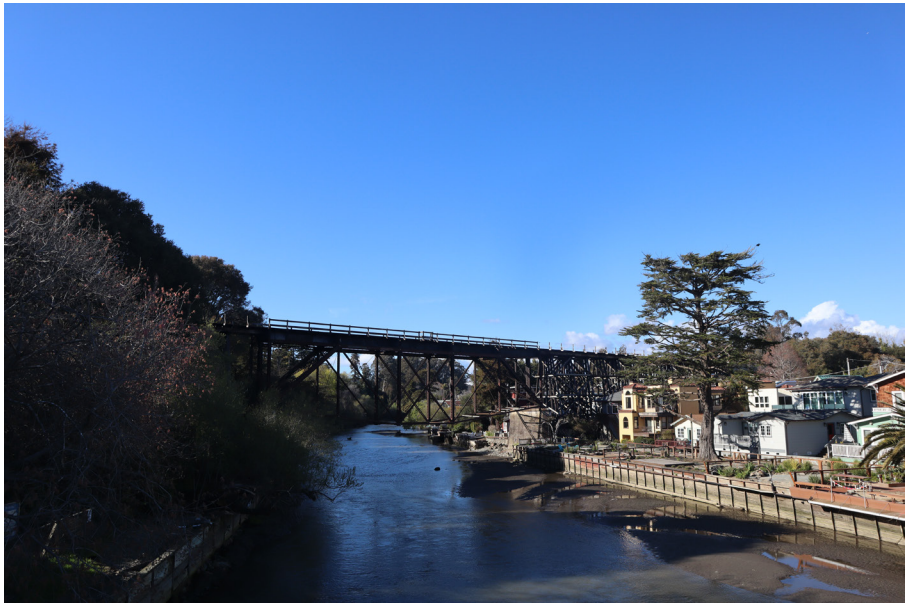
Existing Condition from Key Viewpoint 6, Stockton Avenue Bridge, Looking Northeast. Residential development east of Soquel Creek can be viewed, with Soquel Creek in the forefront and the Capitola Trestle Bridge in the background of the view.
