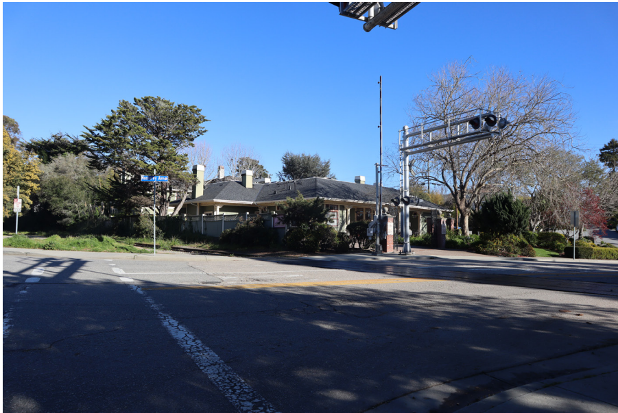
Existing Condition from Key Viewpoint 7, Intersection of Monterey Avenue and Park Avenue, Looking Southeast. This view shows the rail corridor as it extends eastward across Monterey Avenue and continues adjacent to dense vegetation and mature trees along Park Avenue. One tree would be removed from this view, located in the photograph's left background, to the right of the rail corridor.
