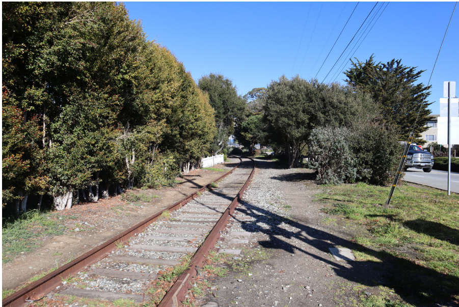
Existing Condition from Key Viewpoint 4, Intersection of Portola Drive and 47th Avenue, Looking East. This view shows the rail corridor as it extends east, adjacent to dense vegetation and mature trees. Several trees would be removed from this view, located in the background to the right of the rail corridor.
