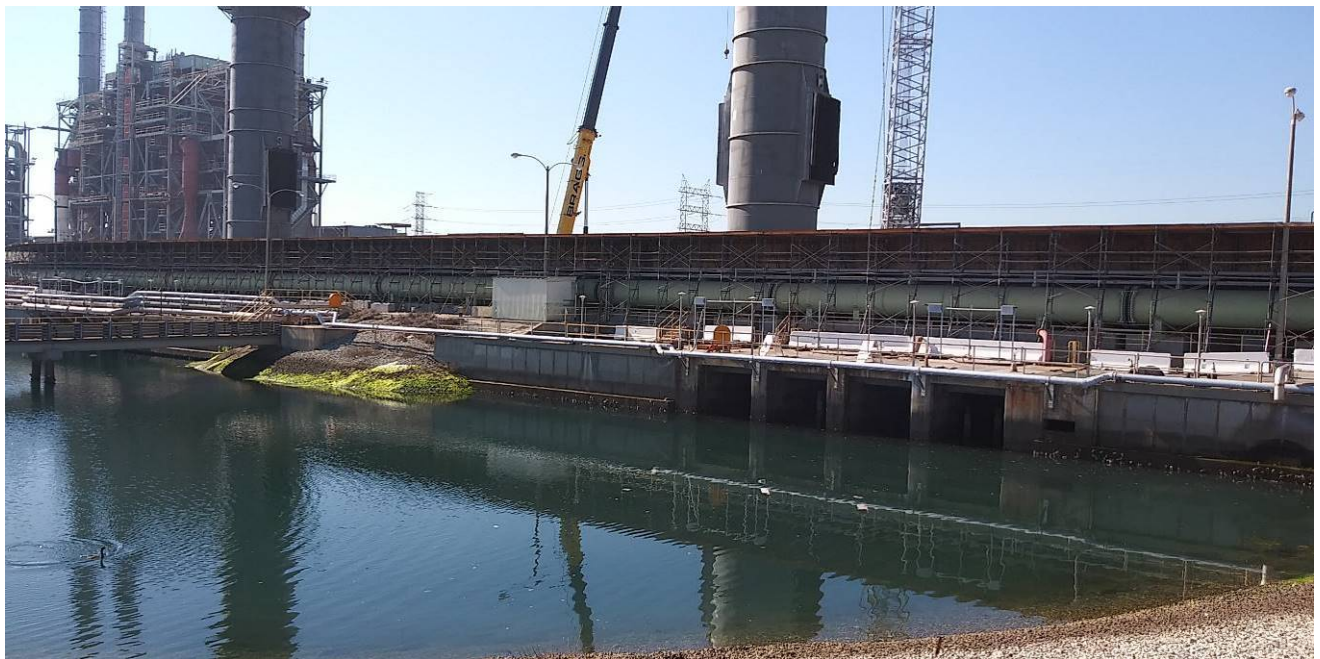
Photo 2. Southeast-facing view of proposed location for the new cooling tower on other side of wall. Haynes Intake Channel in foreground with demolished Unit 4 and Unit 5 stacks in background.
