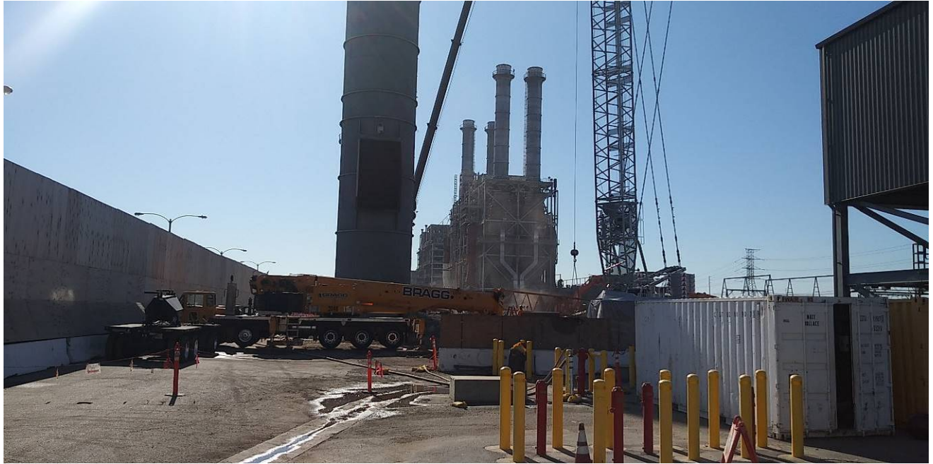
Photo 1. South-facing view of demolition of Units 3 and 4.
