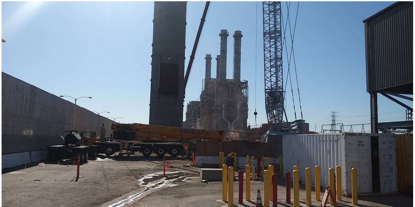
Photo 1. South-facing view of demolition of Units 3 and 4.
