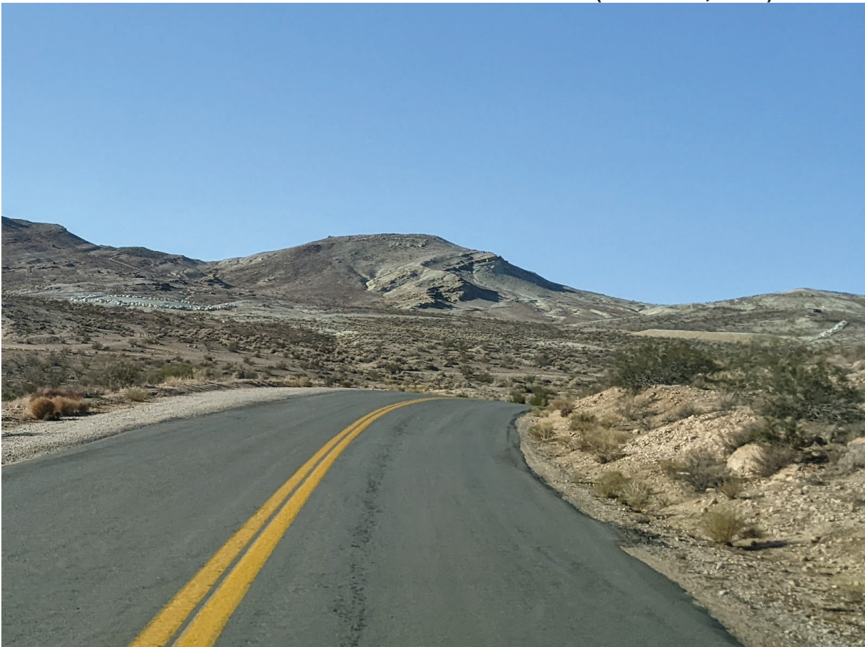
Mojave Tropic Rd adjacent to southeast boundary of project site looking north. Note rising and falling terrain and blind corner. The recently constructed access road intersects just beyond the hill so not in sight of northbound drivers.
