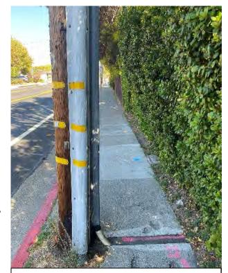
Looking north on Tamal Vista Boulevard adjacent to the Project Site: the width of the existing walkway is reduced to just over 3 feet in multiple locations, due to utility poles placed within the walkway.
