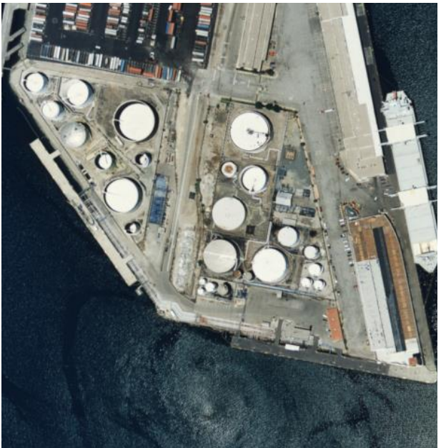
Figure 51: Berths 150-151 as it appeared in 2001: Further reconfiguration of tanks in tank farm. USCB Library.
