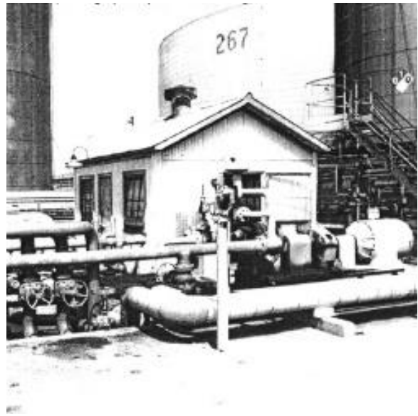
Figure 19: Pump House 2, as it appeared in 2000. Jones & Stokes.
