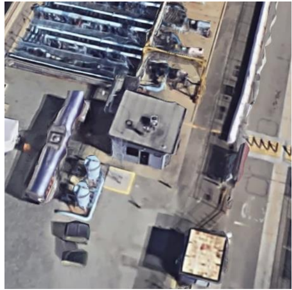
Figure 9: Aerial view of Substation, view looking north. Google Maps.
