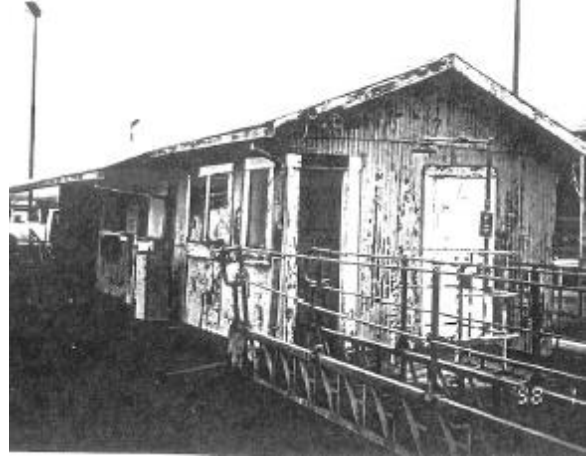
Figure 26: Dock Shed 2, as it appeared in 2000. Jones & Stokes.
