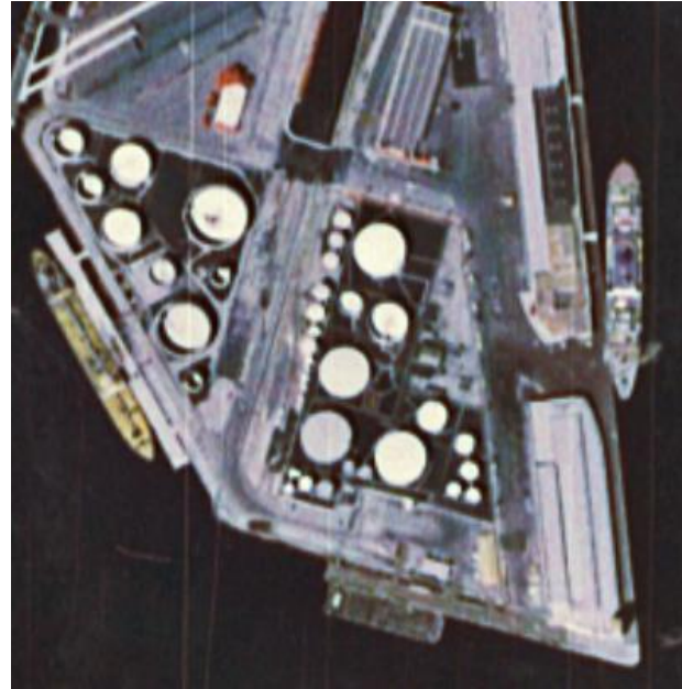
Figure 50: Berths 150-151 as it appeared in 1979: tanks in tank farm reconfigured, Truck Rack constructed. USCB Library.
