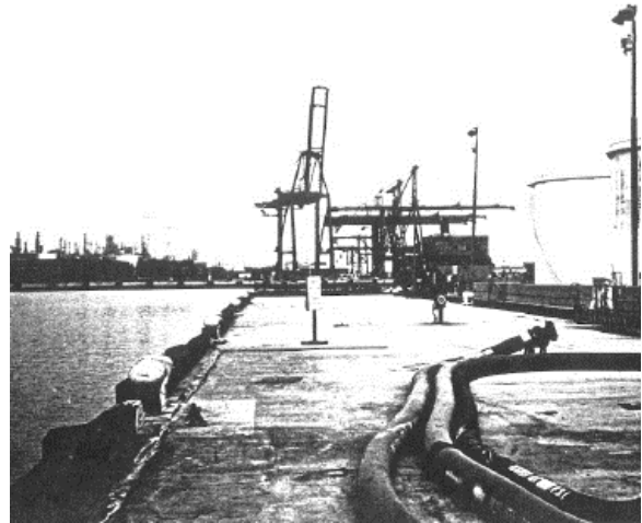
Figure 7: Berth 148-149 Wharf, as it appeared in 2000. Jones & Stokes.
