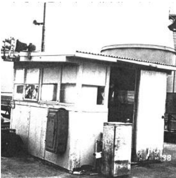
Figure 10: Dock Shed 1 as it appeared in 2000. Jones & Stokes.
