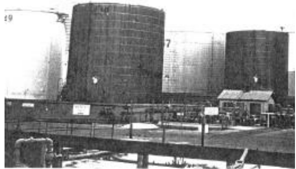
Figure 15: East Tank Farm, as it appeared in 2000. Jones & Stokes.
