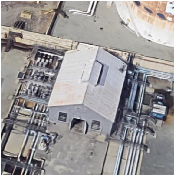
Figure 16: Aerial view Pump House 1, view looking west. Google Maps.
