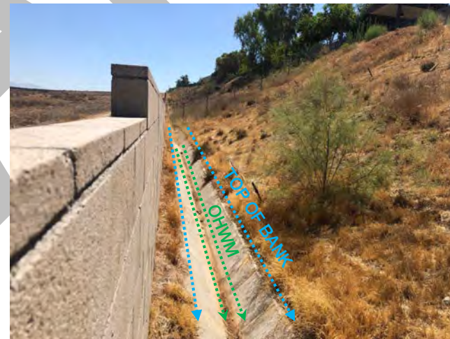
Photo 28. Upstream view of ODP 5 and view of WDP 2, facing east, within NWW-7A1. The OHWM was primarily defined by water staining. WDP 2 met the hydrology parameter; however, WDP 2 did not meet the hydrophytic vegetation or hydric soil parameters (33.898441, -117.313517). August 6, 2021.
