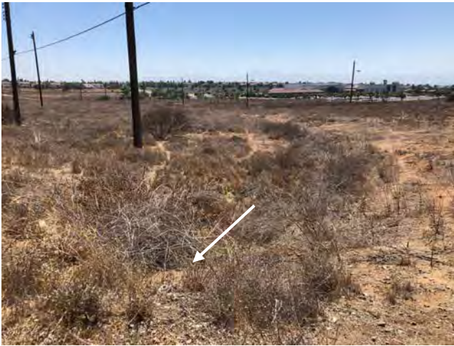
Photo 17. View from culvert (white arrow) that likely historically provided flows to AD-2, facing west (33.903271, -117.310931). August 6, 2021.
