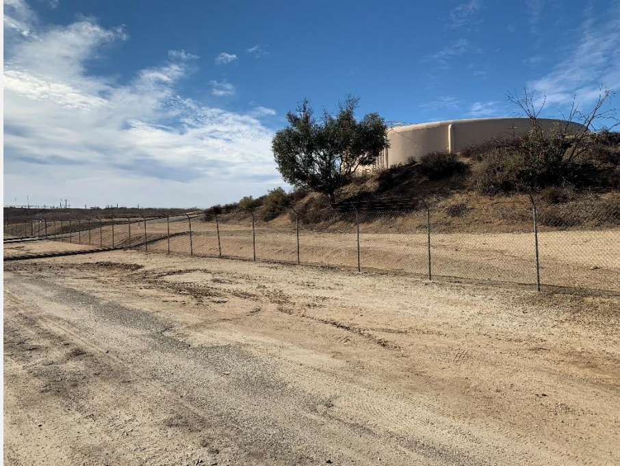
Photograph 3. View of an existing on-site public facility (water tank) located at the terminus of Vista Grande Drive. Photograph taken facing southwest standing just inside of the Vista Grande Drive paved road terminus.
