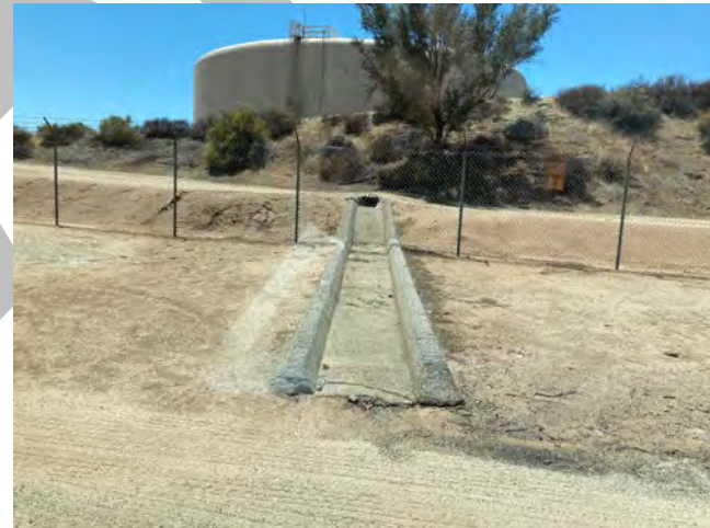
Photo 4. View of Ditch (D-)1, facing west (33.912686, -117.309622). July 28, 2021.
