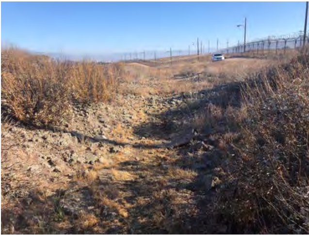
Photo 13. Downstream view of NWW-4 from the culvert (Photo 12), facing north. Broken asphalt had been placed within a portion of the drainage, likely to slow/dissipate flows. NWW-4 exhibited a faint break in slope and change in vegetation cover (33.904788, -117.311987). August 6, 2021.
