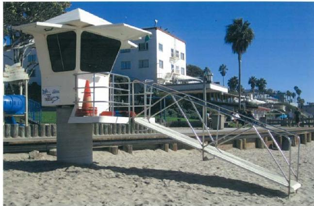
**Photo #2:** Example permanent LOT on pier foundation. Proposed Moss Street LOT similar but ramp replaced with folding stair accessory.
