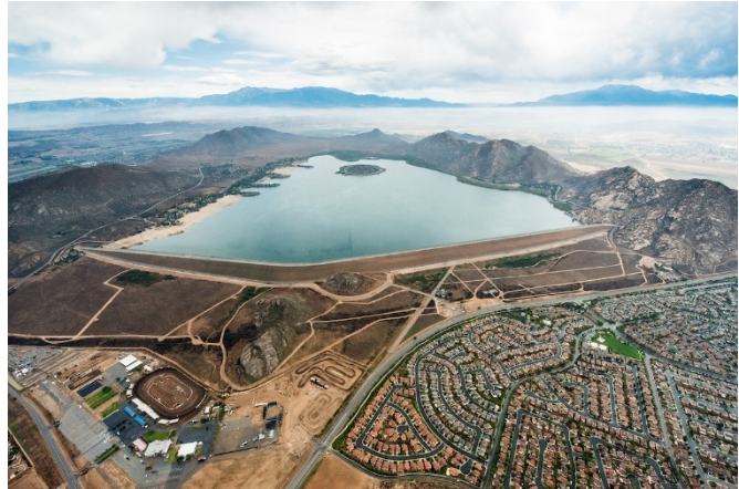
An aerial view of Lake Perris and Perris Dam. Source: DWR
