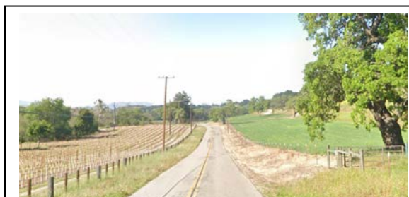
Future uses and related development enabled under the proposed Project would primarily be accessed via the existing County-managed rural road systems such as Foxen Canyon Road, which are often relatively low-volume two-lane roads lacking developed curbs, gutters, sidewalks or street lights.
