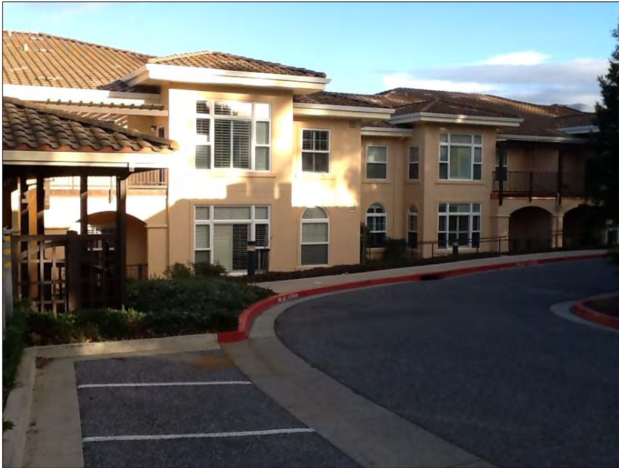
Photograph 10: Apartment building, camera facing west, February 16, 2021.
