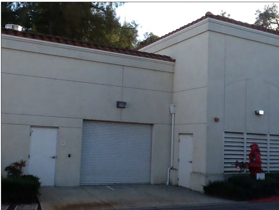
Photograph 14: View of Utilities and Garage Building, camera facing east, February 16, 2021.
