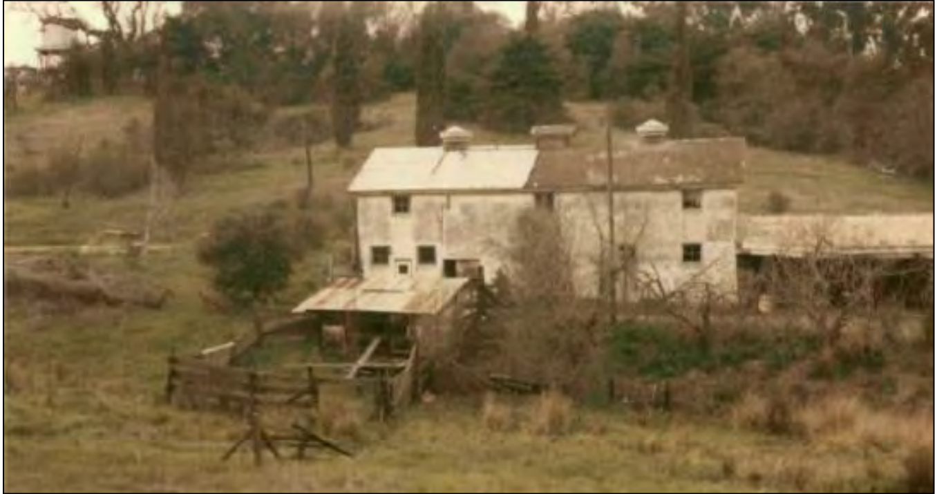
Plate 6: Circa 1984 photograph of the southern cow barn (no longer extant). This barn and the barn to the north were demolished between 1987 and 1991 and are shown as only foundation pads on the 1994 Site Plan below. (Source: Attributed to Letter to Mike Flores, Secretary of Heritage Preservation Commission from illegible author, 1984 June 25)
