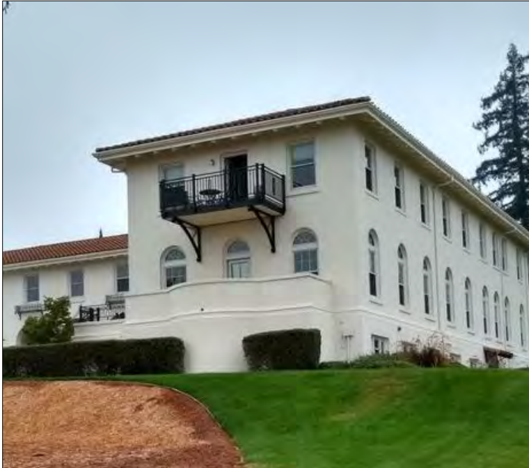
Photograph 5: North and east elevations, camera facing southwest, October 7, 2020.
