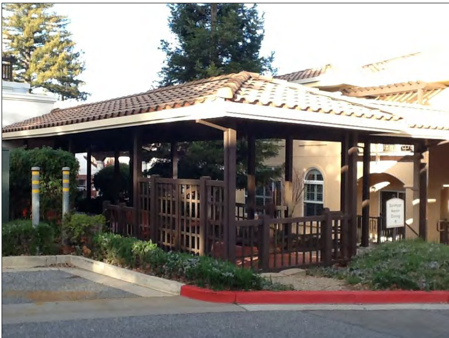
Photograph 11: Apartment building cover walkway, camera facing northwest, February 16, 2021.
