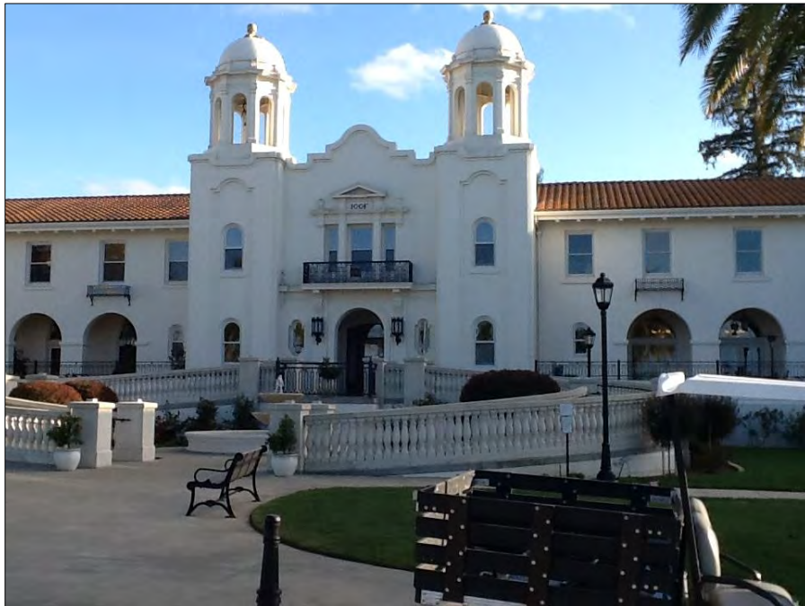
Photograph 4: Detail view of facade, camera facing south, February 16, 2021.
