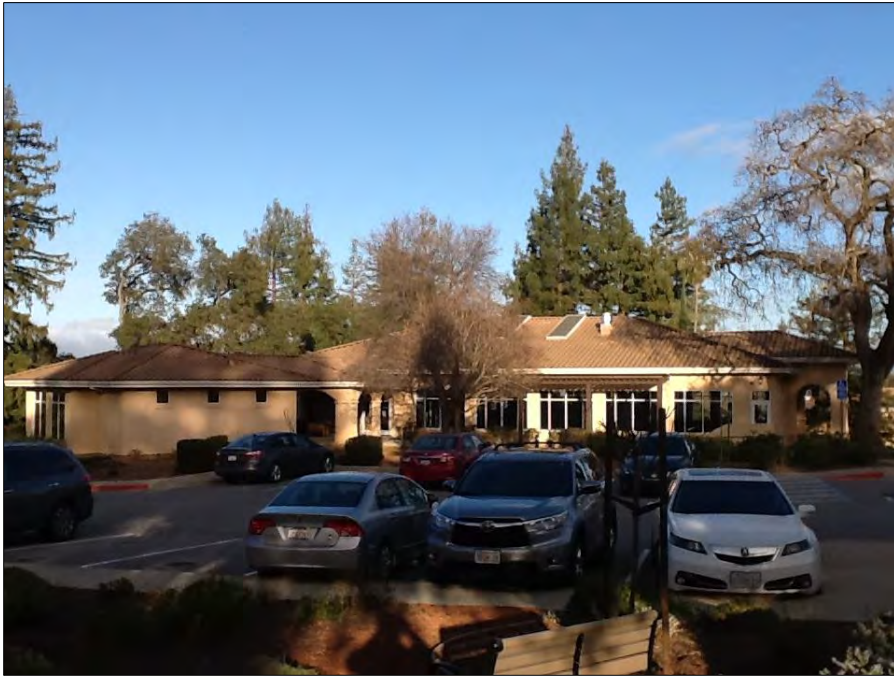
Photograph 12: Fitness Center, camera facing west, February 16, 2021.
