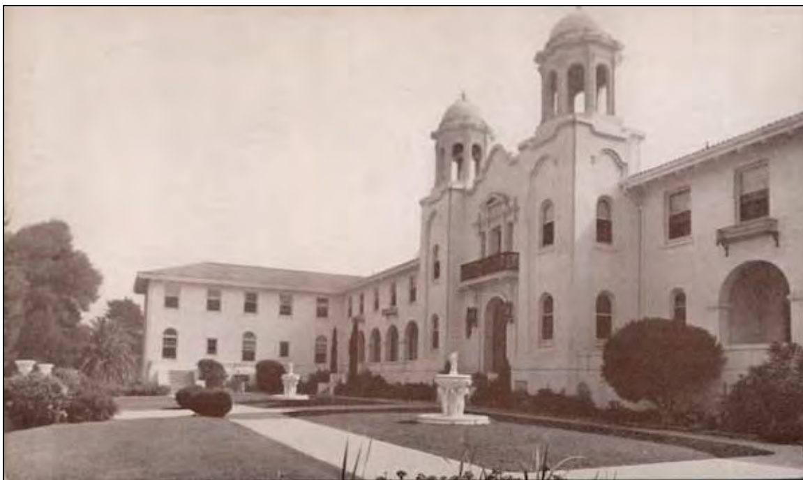
Plate 13: Undated photograph showing the small fountains on the original terraced landscape. This entire area was graded in 2003 with new landscaping and the large fountain and ramps installed in 2004. (Source: https://www.cardcow.com/738786/saratoga-california-odd-fellows-home/ ).
