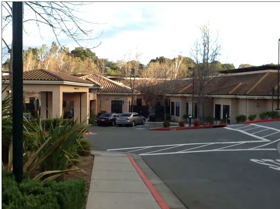
Photograph 9: Health Center entrance, camera facing southwest, February 16, 2021.
