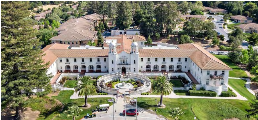
Saratoga Retirement Community-Manor Building after the 2005 construction.
