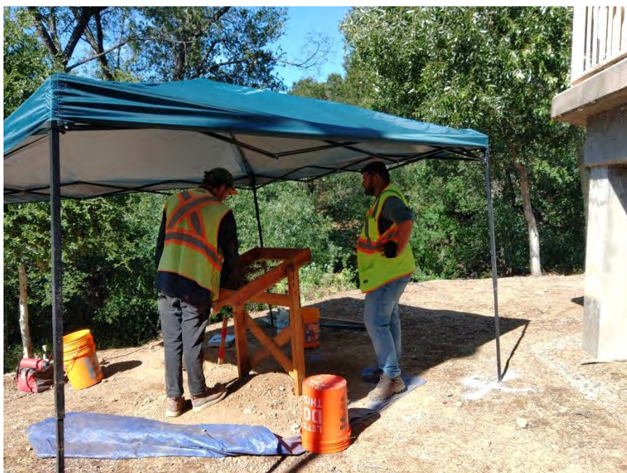
Photograph 7: Excavation overview at STP1 location, view east-northeast. 6/09/2022.
