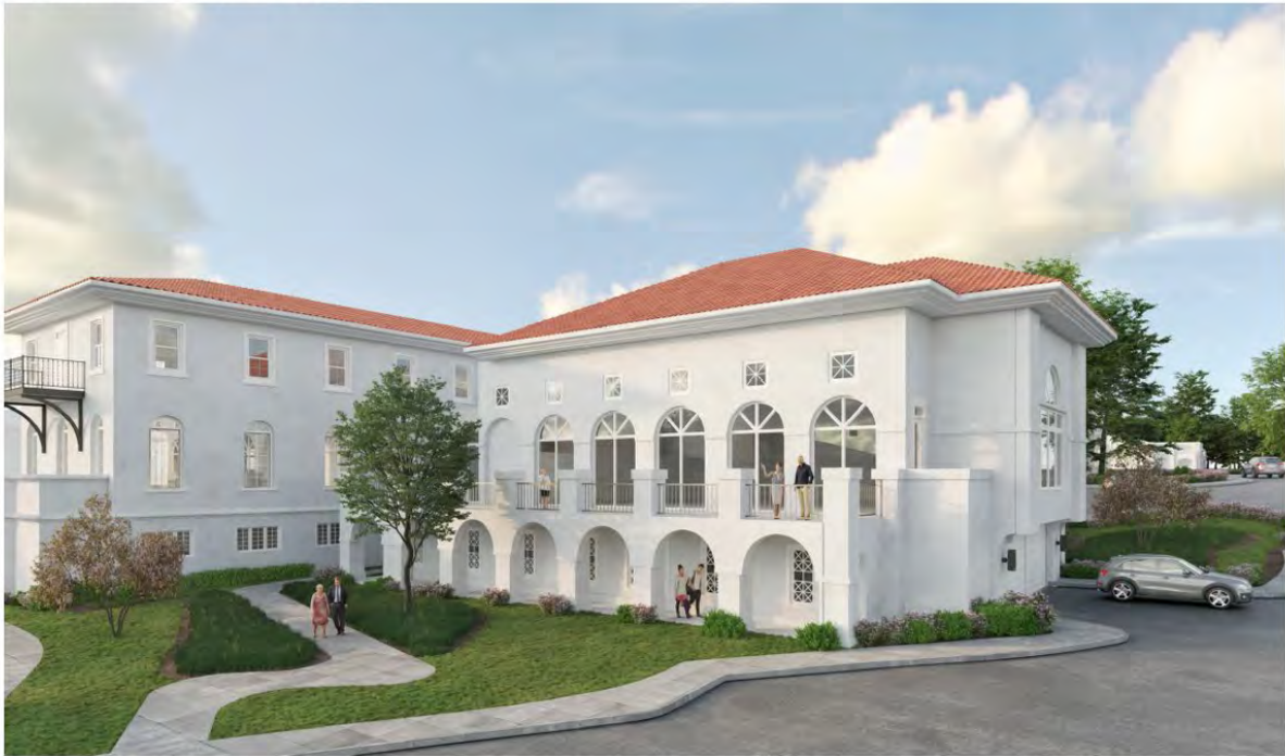
ANKROM MOISAN ARCHITECTS, P.R.S. AND I/O/F:2 1 SARATOGA RETIREMENT COMMUNITY INDEPENDANT LIVING & AUDITORIUM EXPANSION
