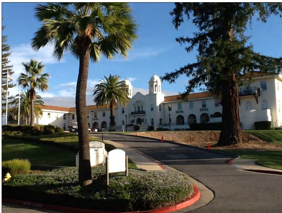
Photograph 3: View of roadways and landscaping, camera facing southwest, February 16, 2021.
