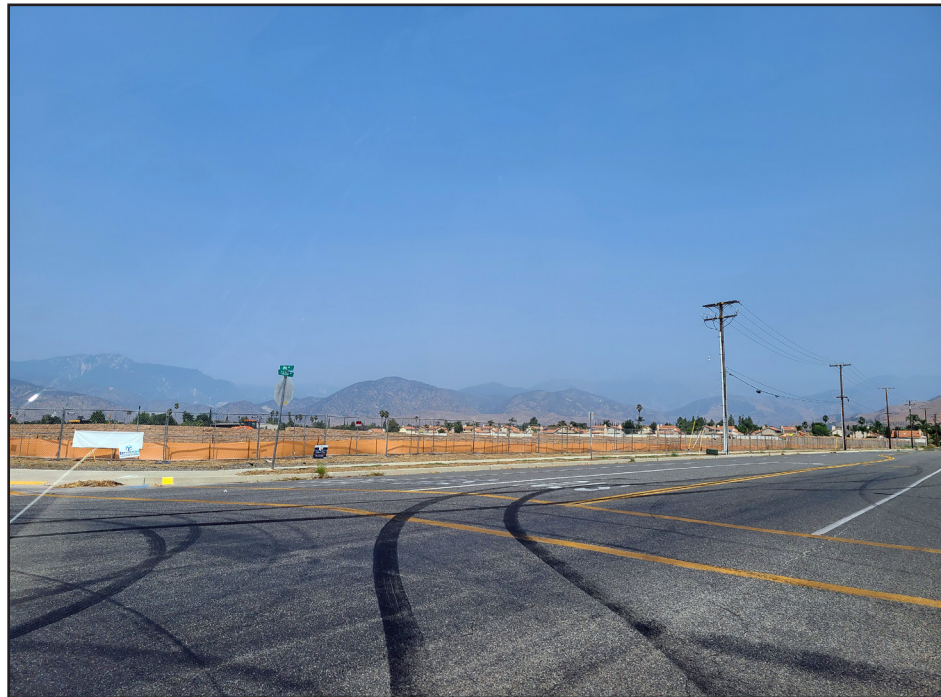
View 5: From the intersection of Colton Avenue and Opal Avenue, looking northeast at the active construction site north of the project site and the residential neighborhood to the northeast of the project site.
