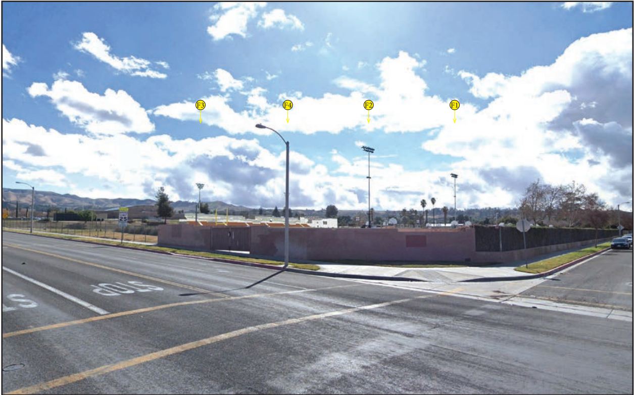
Photo 2. View of project site looking southeast.
