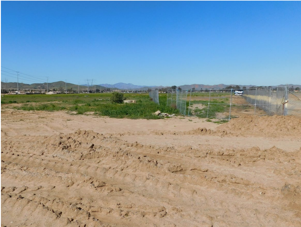
Photograph 5: From the eastern boundary of the project site at Barnett Road looking west across the eastern portion of the site.
